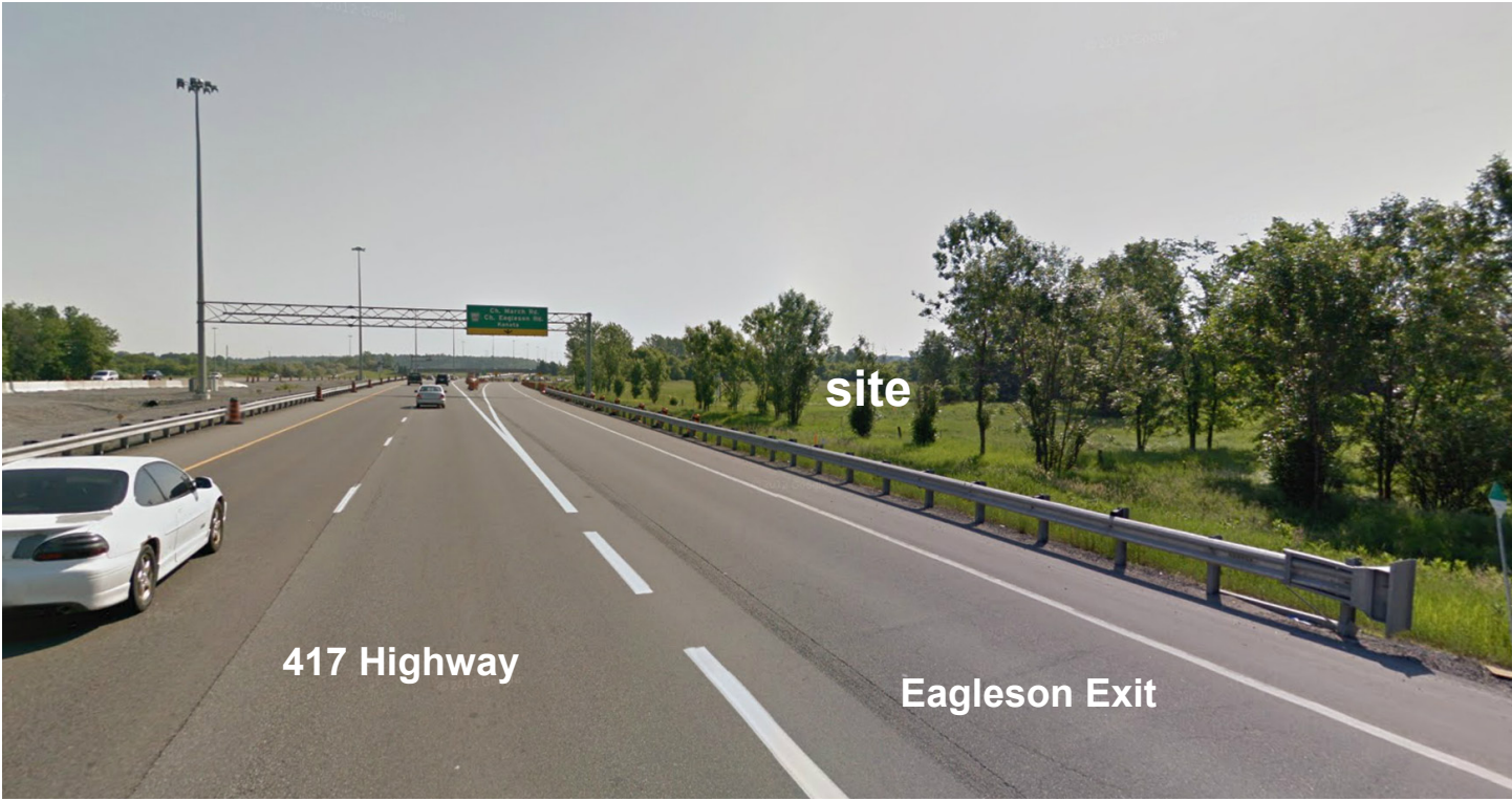
Fig. 3 - Image | View from 417 (Eastbound)
