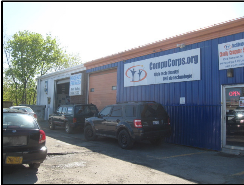
Photograph 1: View of the north side of the subject structure looking southeast. Photograph illustrates the location the automotive service garage, at the east end of the building, and CompuCorps.
