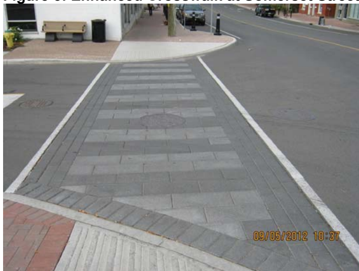
Figure 5: Enhanced Crosswalk at Somerset Street/Breezehill Avenue
