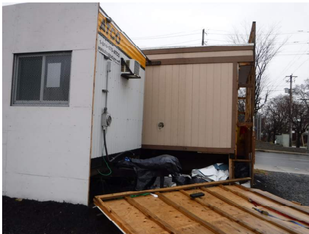
Photograph 3: Southwest corner of the on-site trailers.
