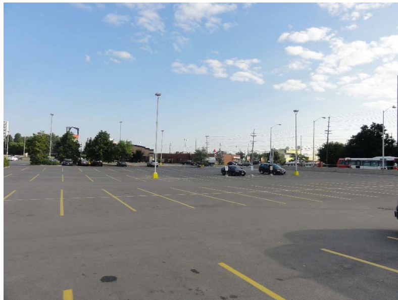
Photo 6 – General view of the asphalt paved parking area on the southern portion of the Site.
