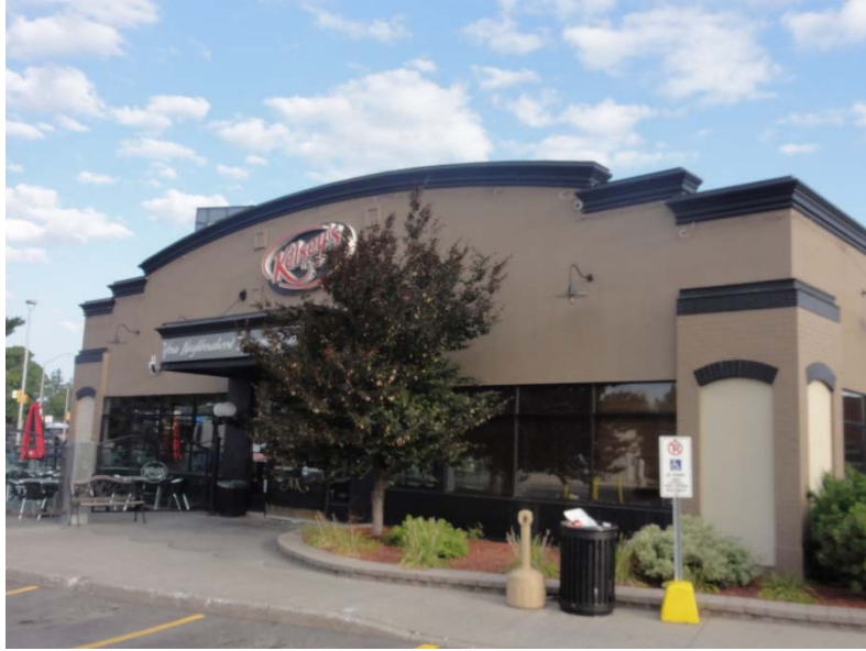
Photo 1 – View of the south elevation of the Site Building, looking northwest.
