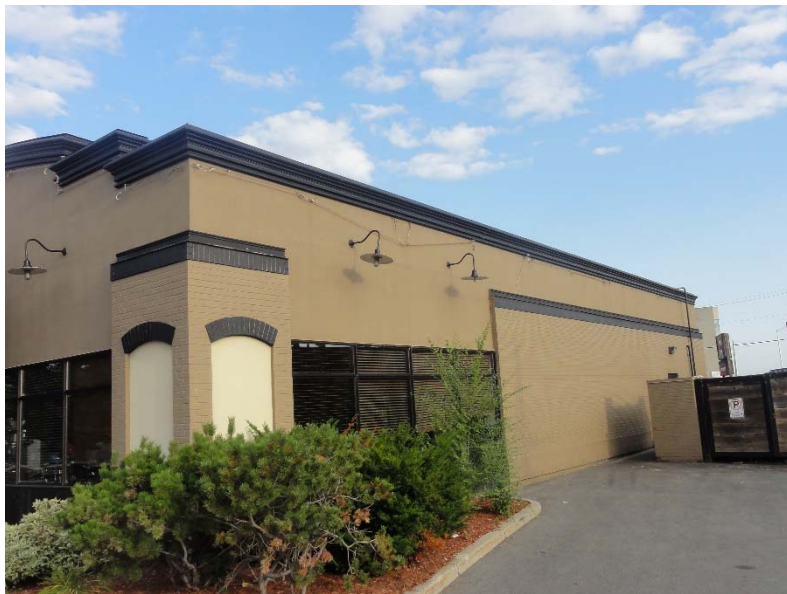
Photo 2 – View of the east elevation of the Site Building, looking northwest.
