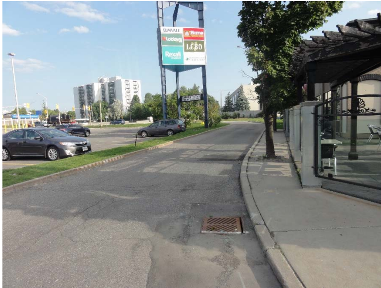
Photo 3 – View of the asphalt paved driveway off of Smyth Road that provides access to the Site.
