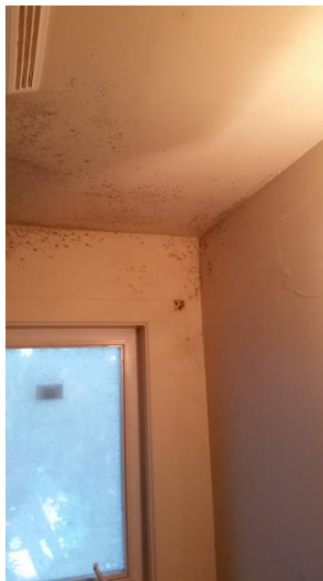
Photo 8: Interior, presence of mold on walls.
