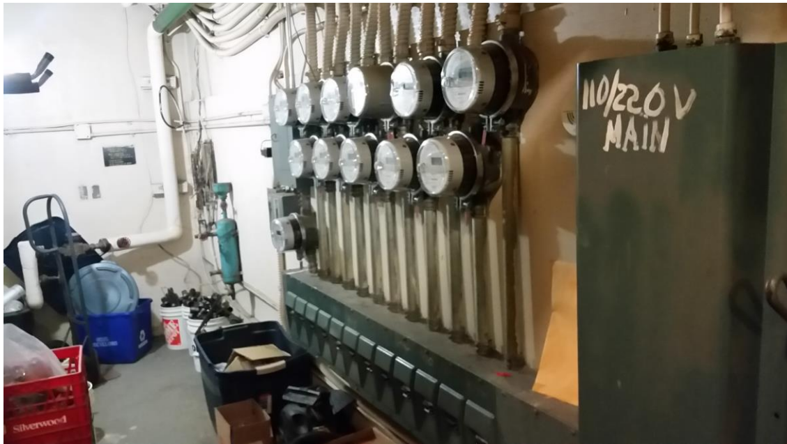
Photo 15: Mechanical room hydro meters.
