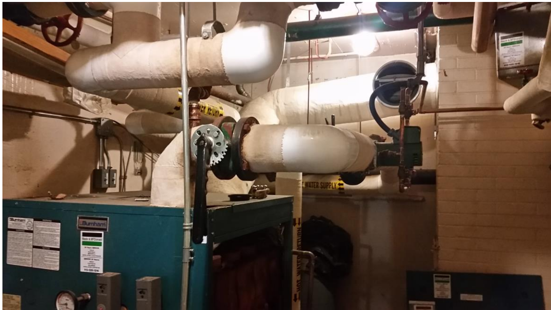
Photo 14: Mechanical room steam lines.
