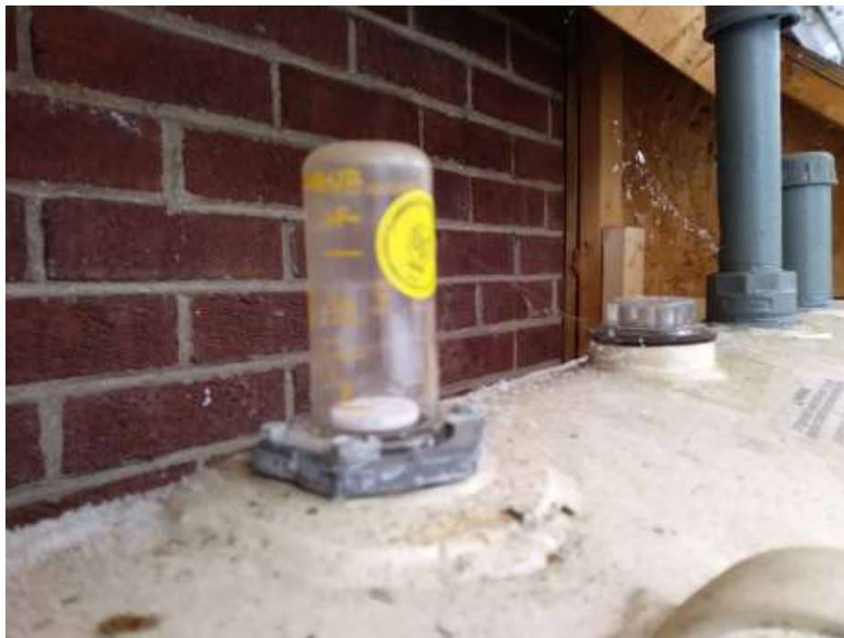
Photograph 3. Fuel level gage on furnace oil tank (reads empty)
