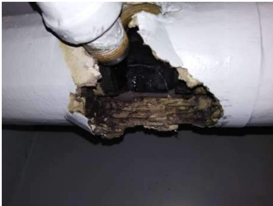
Photograph 11. Burst pipe with possible asbestos insulation
