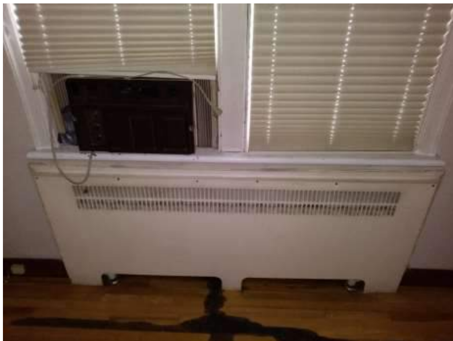
Photograph 9. Window air conditioning unit and water leak from radiator
