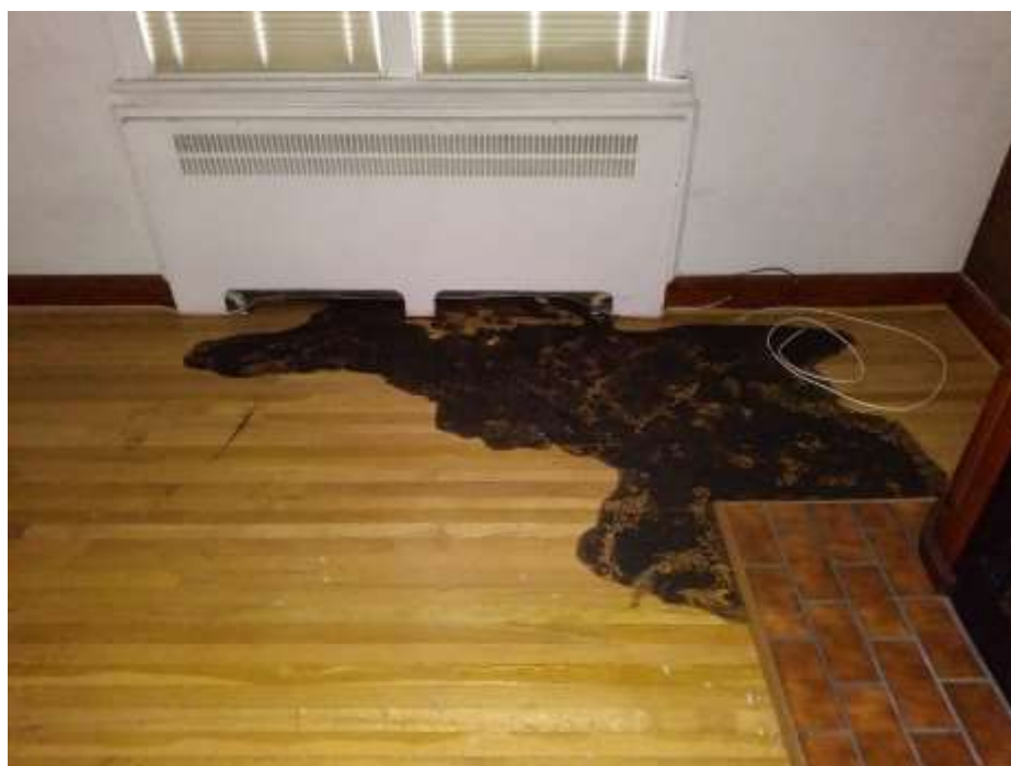
Photograph 8. Water leaking from stream radiators due to burst pipes, typical of majority of radiators in residence.
