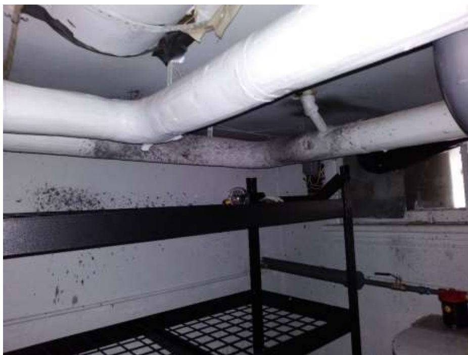
Photograph 6. Typical burst pipe and water damage (observed throughout basement)
