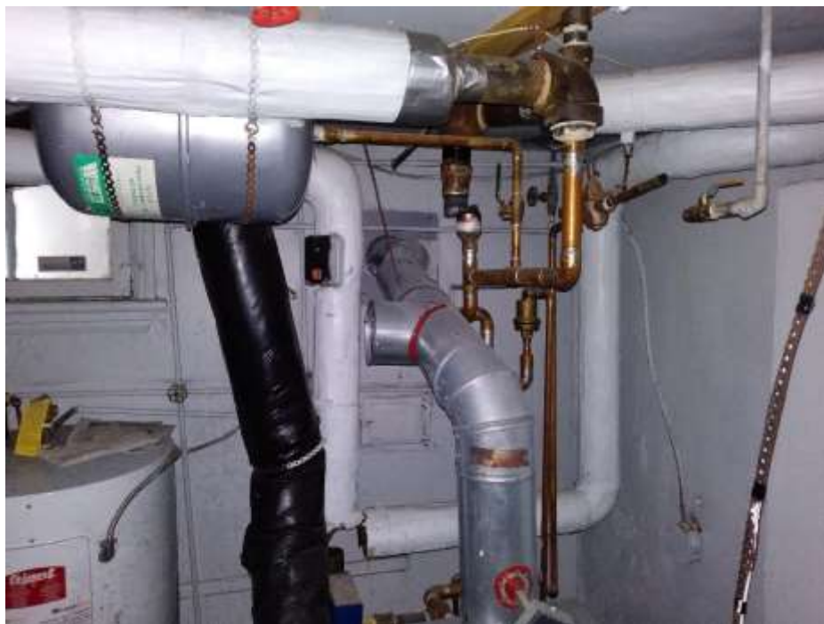
Photograph 5. Interior of residence basement, showing oil furnace boiler and multiple frozen/burst pipes
