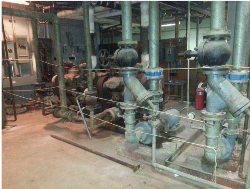
Photo 37 – Compressors and pump associated with the historical cooling units used in the grocery store (out-of-service). Old Carrier units.
