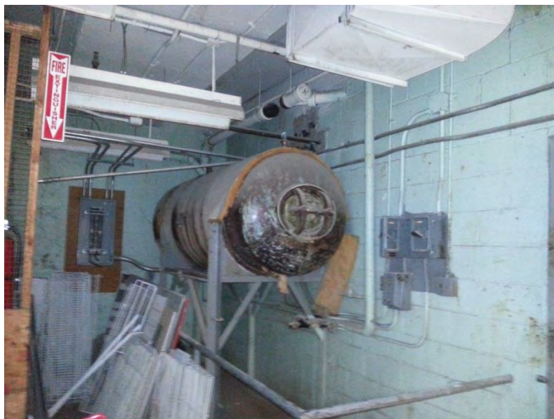
Photo 33 – Air tank reported to be associated with the out-of-service boilers before switching to natural gas. Also, old fluorescent lights shown.
