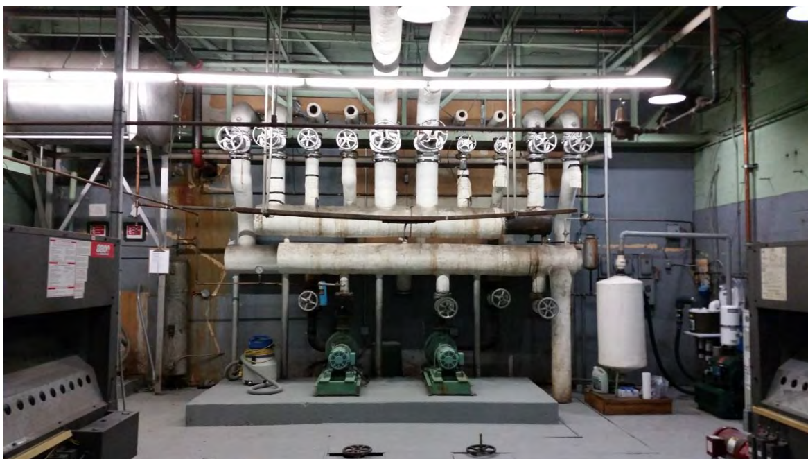
Photo 81 – Boiler room. Former boilers have been replaced with natural gas boilers. Much infrastructure from the original boilers has been retrofit to work with the newer natural gas boilers. Equipment for the dentists office is also located in the boiler room.
