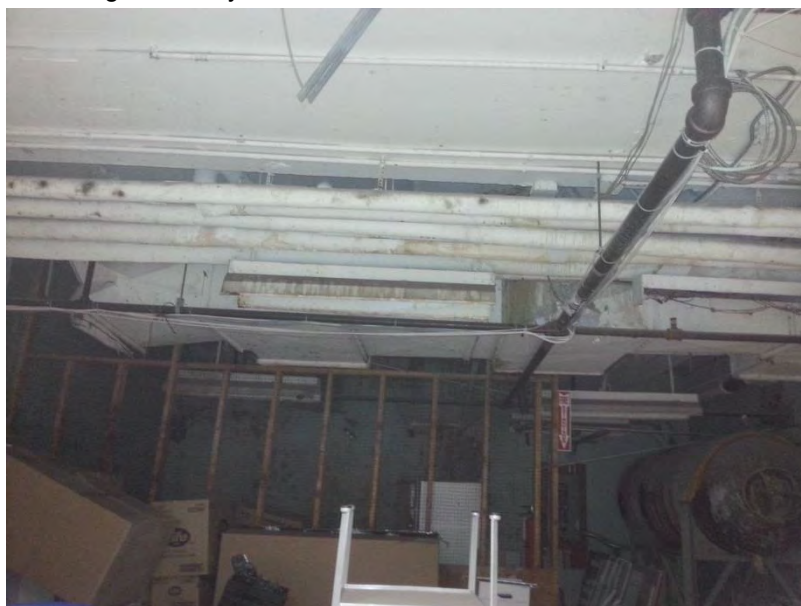
Photo 32 – Asbestos insulation on pipes.
