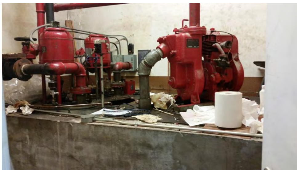
Photo 66 – Sump pit in Cozy Coverings back room. 2 working electrical pumps and 1 out-of-service gas powered pump.
