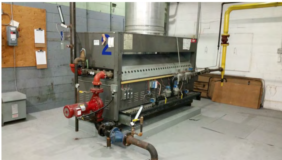
Photo 85 – Natural gas boiler.
