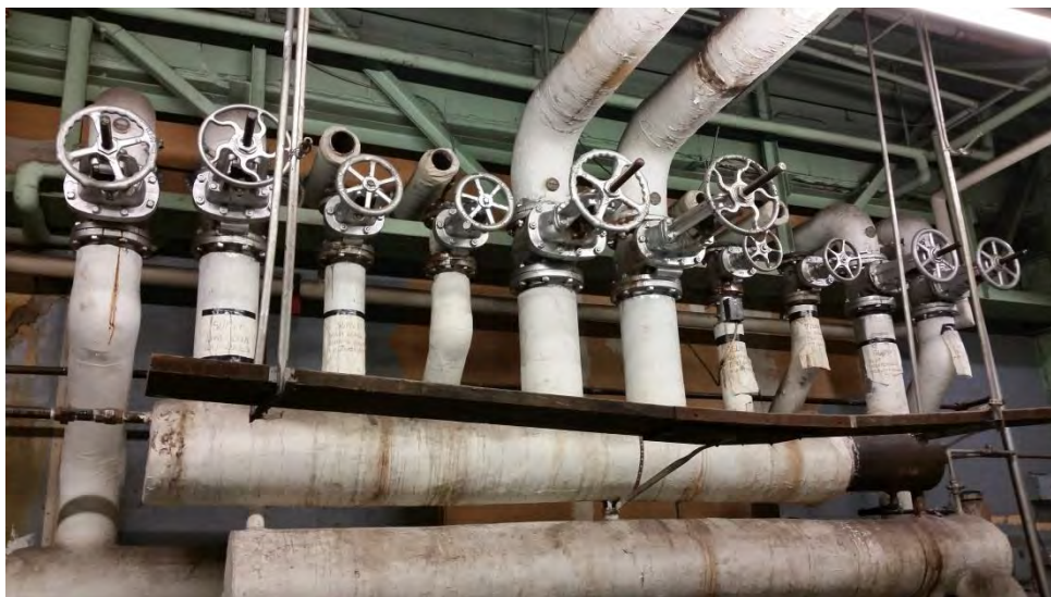
Photo 83 – Valves controlling air flow to some tenant spaces and the mall corridors.
