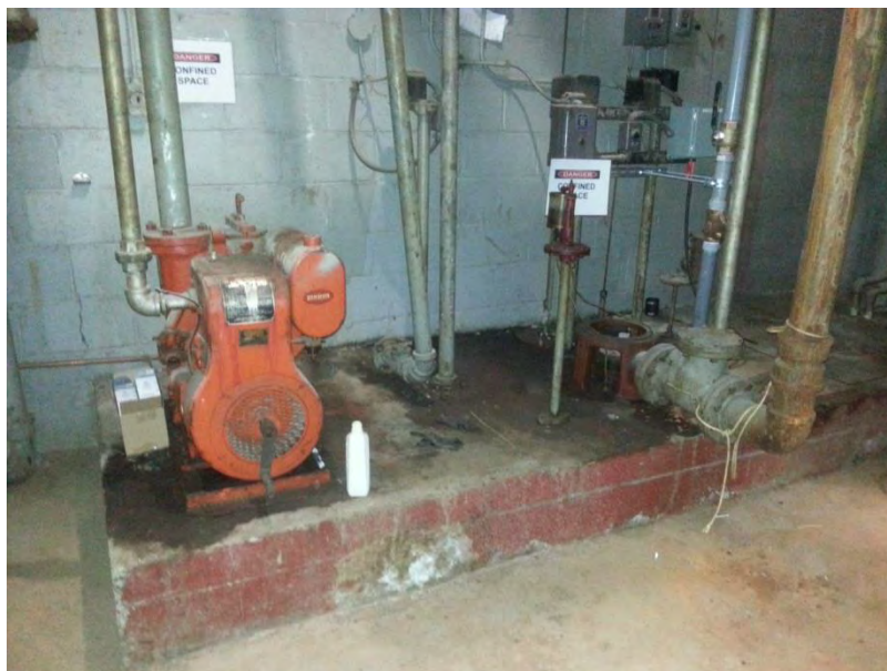
Photo 35 – Sump pump in basement.
