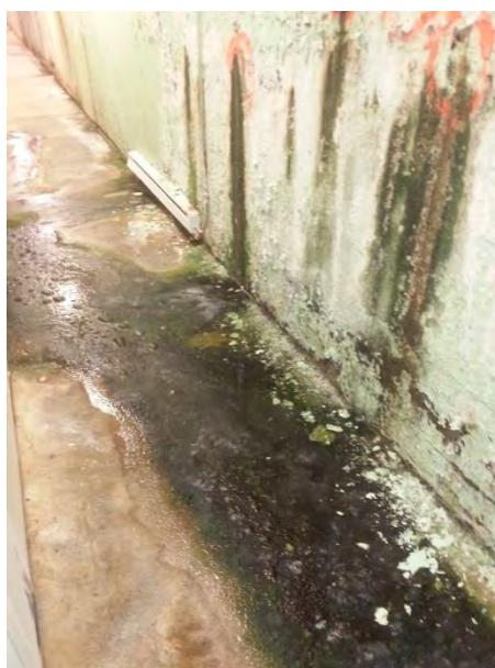
Photo 48 – Significant mold and water damage in the basement hallway. Water was coming in through the concrete foundation.
