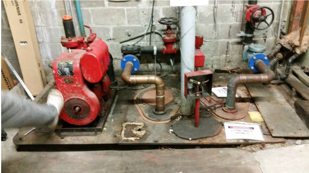
Photo 103– Sewage collection pumps. Sewage from the eastern part of the building is collected in the pit and pumped to the City of Ottawa sewer.
