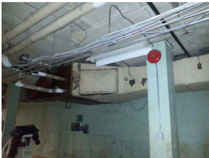
Photo 40 – Existing forced air infrastructure in the basement (out-of-service) and asbestos covered pipes. Also shown are older style fluorescent bulbs.
