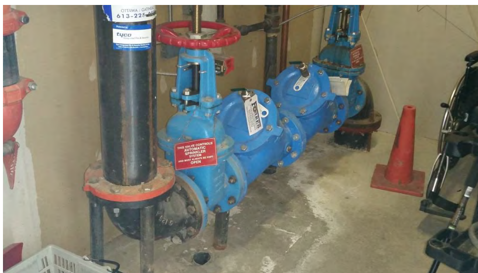
Photo 88 – Sprinkler risers.
