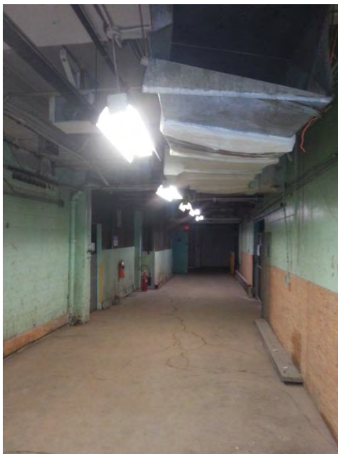
Photo 31 – Basement hallway. No lighting retrofit. Asbestos insulation is present on pipes and paint is original to the former Steinberg's Grocery Store.
