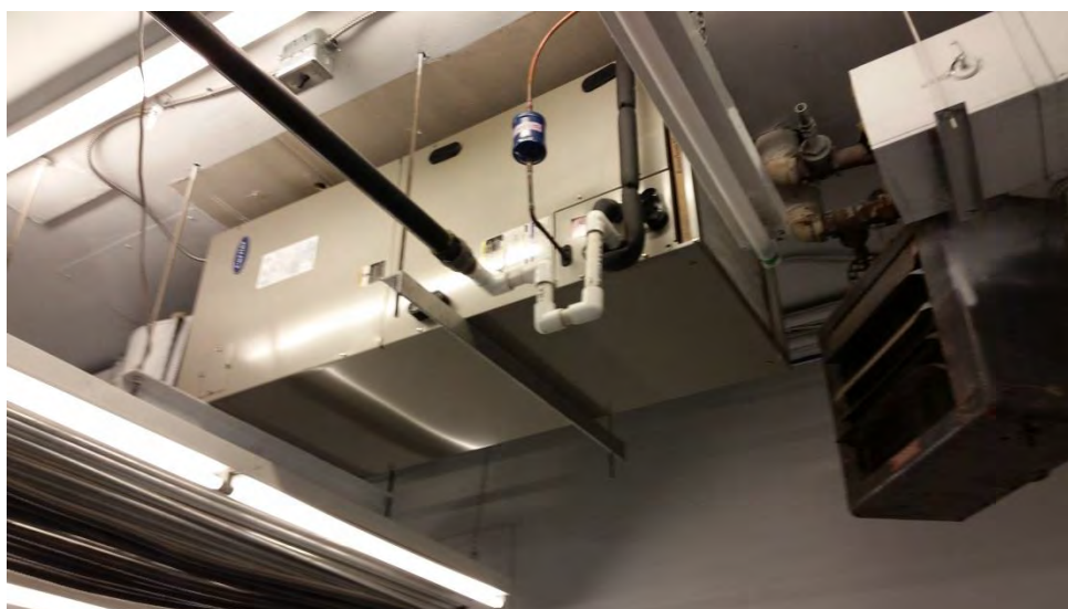
Photo 70 – Indoor portion of roof mounted HVAC equipment. All natural gas powered and the majority of tenants are responsible for their own maintenance.
