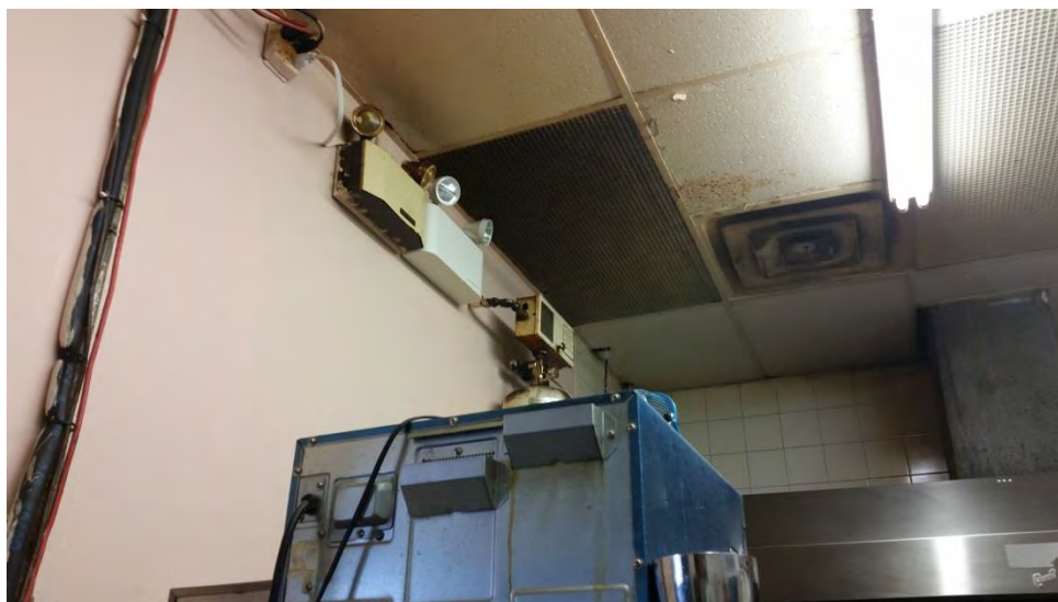
Photo 74 – Staining on ceiling tiles in Rockin' Johnny's Restaurant.
