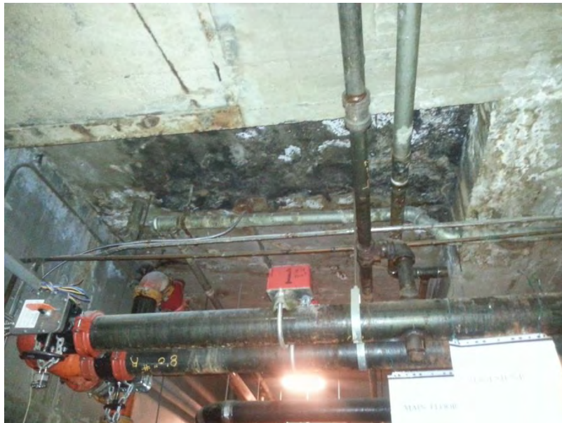
Photo 38 – Sprinkler system infrastructure and mold on the ceiling.
