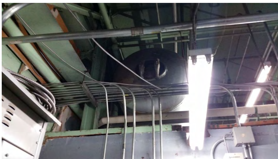
Photo 86 – Air tank. In use with the updated boiler system.
