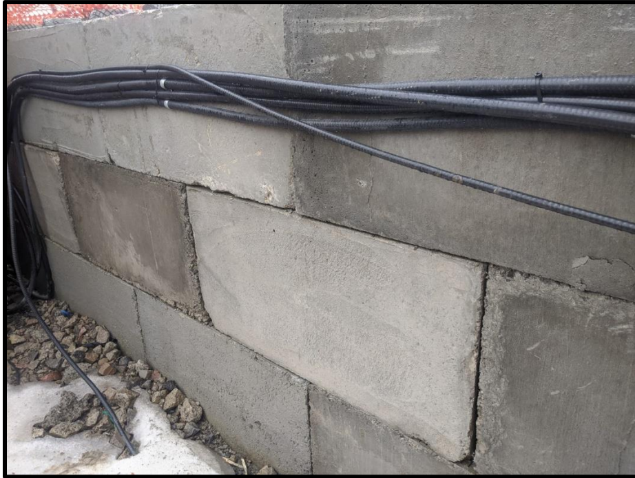
Photo 2: Photo of north face of lower retaining wall. Some soil noted sloughing onto the retained fill from the existing stockpile uphill from the retaining wall.
