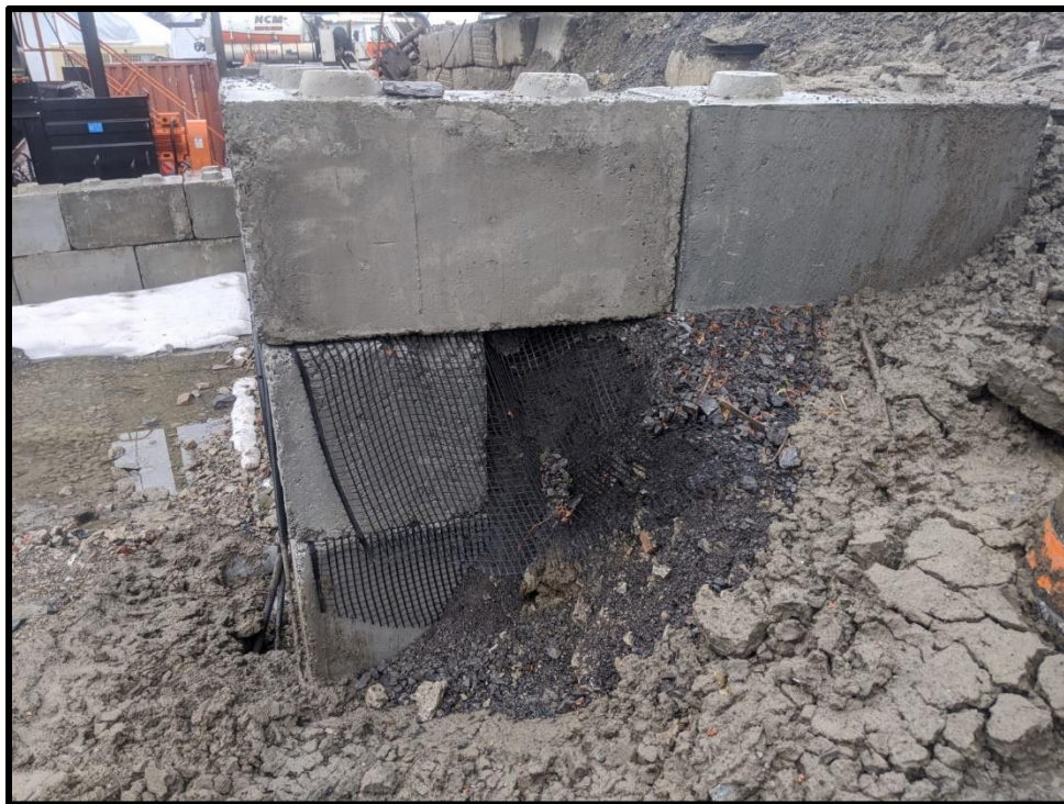
Photo 2: Photo of north face of lower retaining wall. Some soil noted sloughing onto the retained fill from the existing stockpile uphill from the retaining wall.
