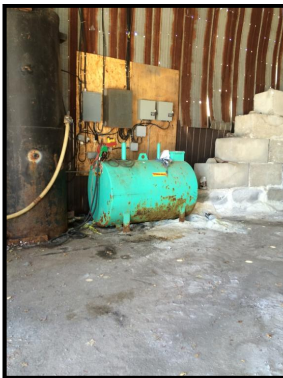
Photograph 12: Aboveground diesel storage tank, located in enclosed portion of building. Note the salt storage area on the right side of the photograph, and one of the steel brine silos on the left side of the photograph.
