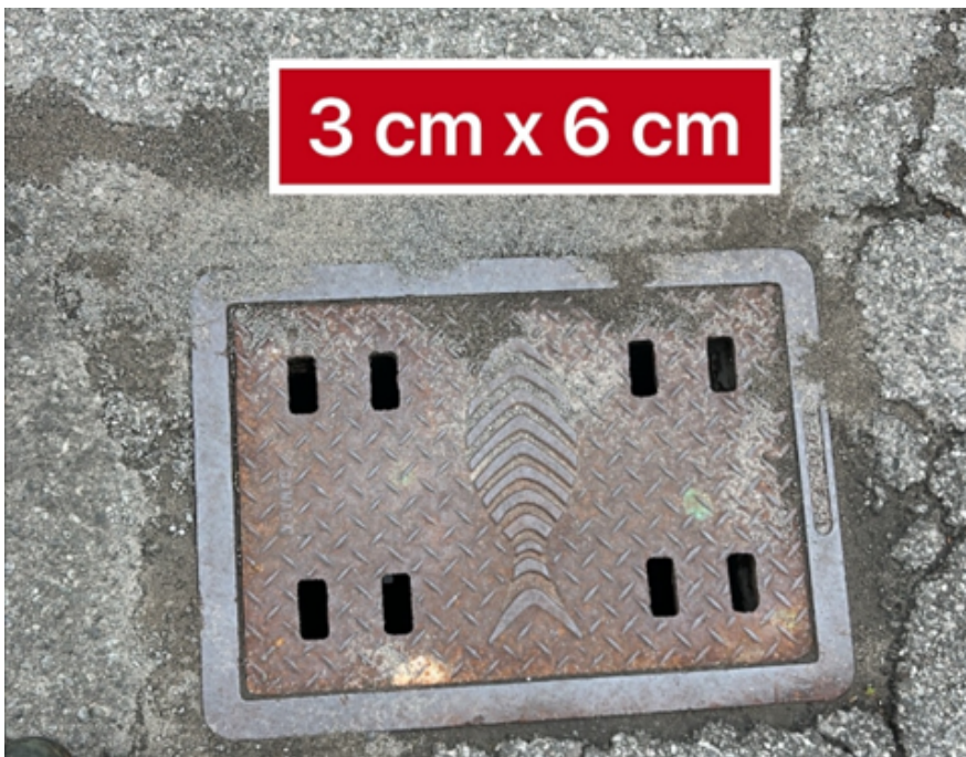
Closeup EX CB 1 (from Site visit) with noted dimensions of openings
