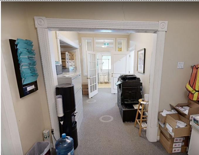
Figure 9 – Ground Floor, existing finishes in the main corridor of the Stone Residence. Note later replacement cased openings.
