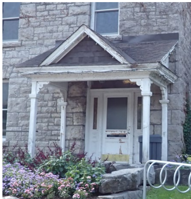
Figure 6: Existing porch on the Stone Residence (Source: RMA+SH architects, 2026).
