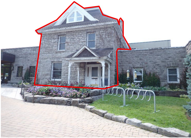
Figure 2 – Portion of building proposed for demolition (red outline), known as the 'Stone Residence'.
