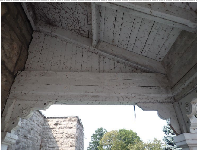
Figure 6 – Wood front porch of Stone Residence. Note decorative fretwork brackets and vines beginning to sprout throughout wood surfaces.
