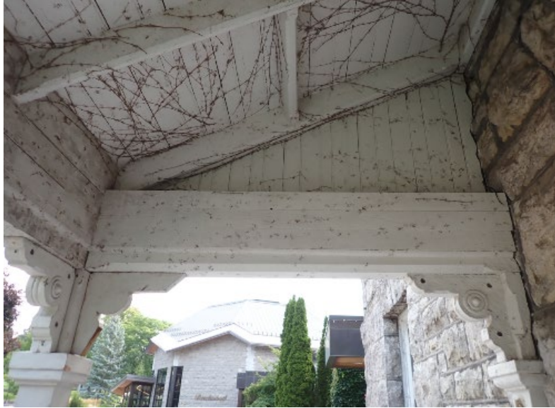
Figure 7: Detail of existing porch with wood ceiling, columns, and fretwork on the Stone Residence (Source: RMA+SH architects, 2026).
