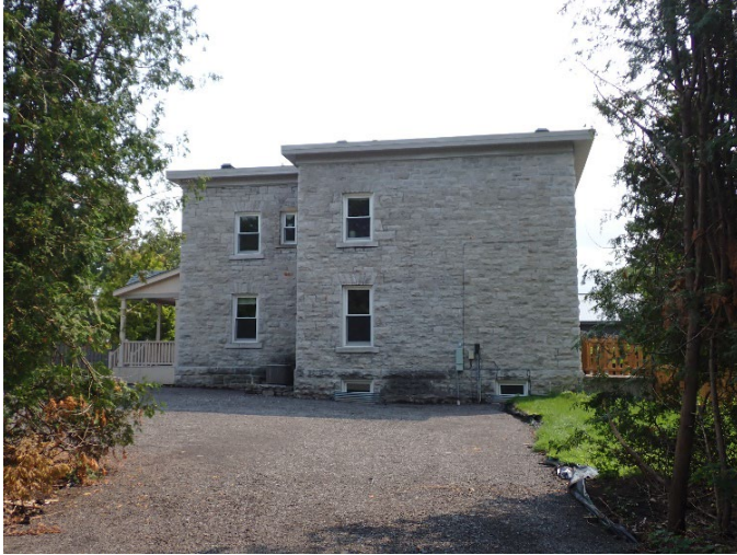
Figure 23 – The original double stone residence (with stone quarried from the site) for gardeners and foreman, contemporary with the Subject Site, currently used for administration.
