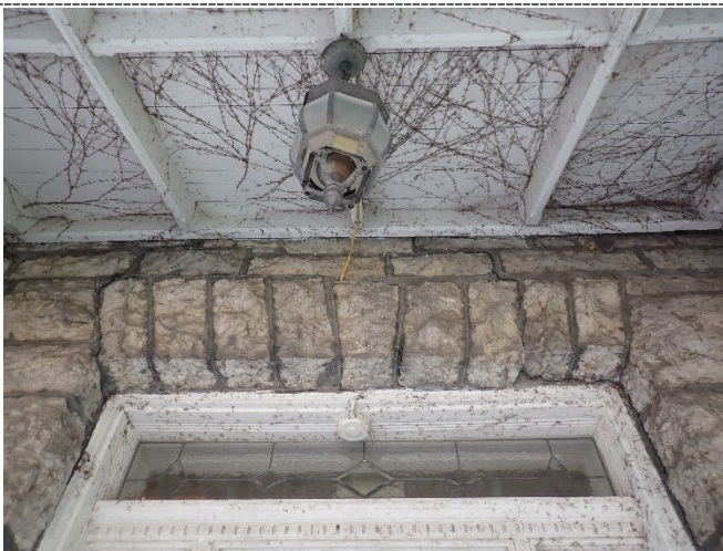
Figure 7 – Wood front porch and transom above door of Stone Residence. Note vines beginning to sprout on both masonry and wood surfaces.
