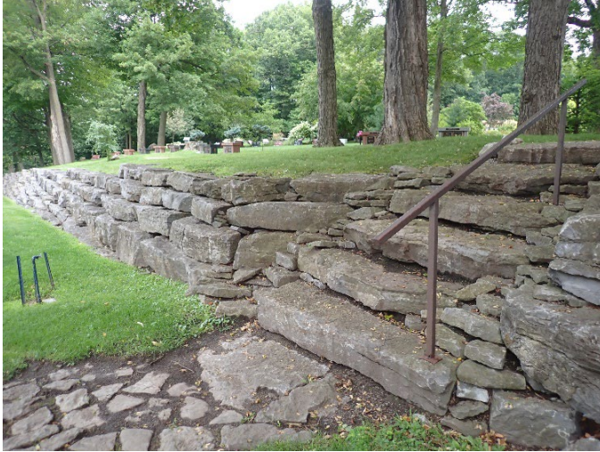
Figure 20 – Limestone stairs and retaining wall (assumed quarried from the site) along southern edge of Botanical Cremation Gardens, lining the main entrance road.
