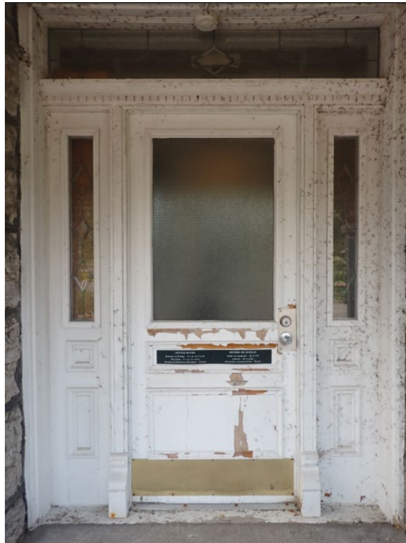
Figure 4: Existing front door on the Stone Residence (Source: RMA+SH architects, 2026).
