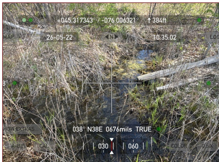
Site Photograph 7: Pocket of standing water.
