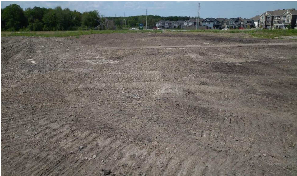
Photograph No. 4: Facing West Across Site to Proposed Building Location from West Edge of Work Area
