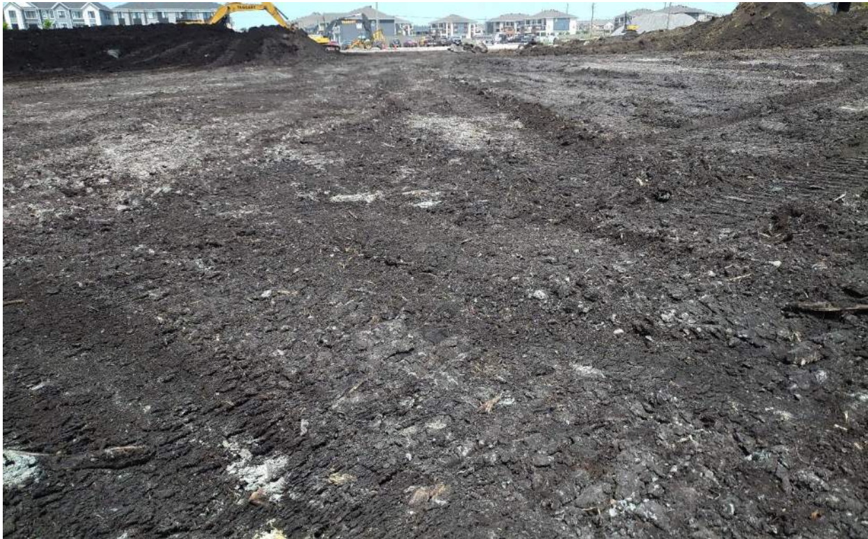
Photograph No. 5: Low Point of Removals Facing North – Fill Material Remaining
