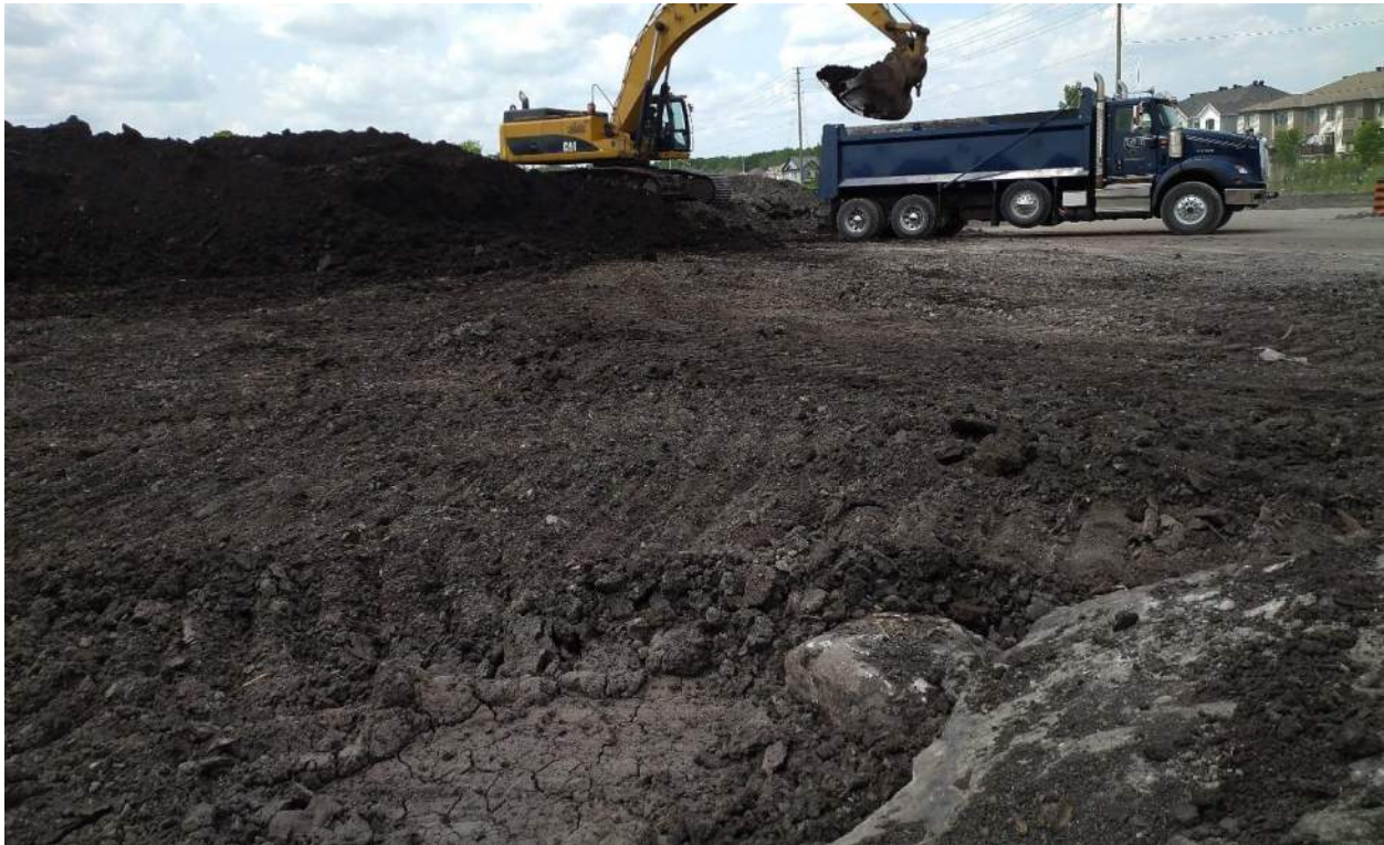
Photograph No. 1: Contractor Loading Topsoil and Removing It Off-Site
