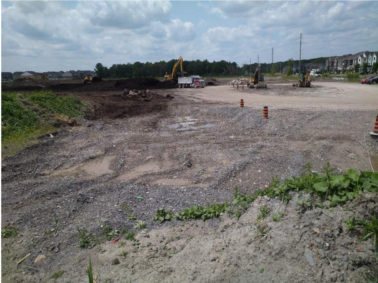
Photograph No. 7: East Edge of Site Facing West
