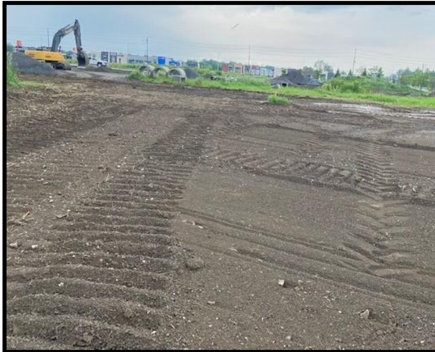
Photograph 8: View of the former construction debris piles location along Limebank Road, facing north.
