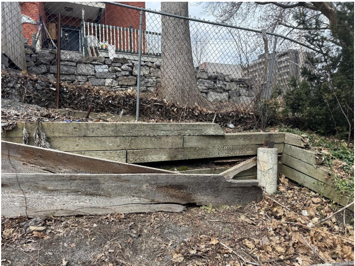
Photo 1: Existing wall by Tree 10, American elm on adjacent property. The new retaining wall will be over 4 m in depth and flush against the property line which is close to the existing fence
