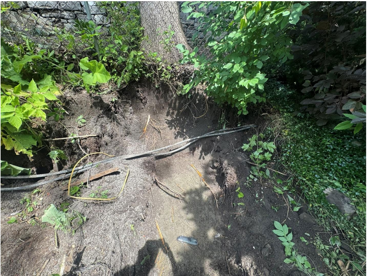
Photo 3: Soil and roots visible after the removal of the wall
