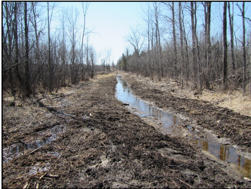
Photo 16 - Realigned northwest swale along the north edge of the site. View looking west, with section of remaining trees to the left, south, and MTO lands to the right, north (April 15 th , 2016)
