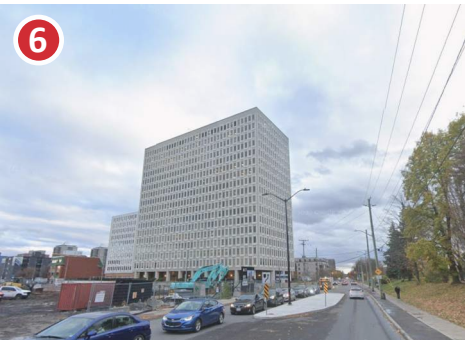
Looking south down N River Rd.
