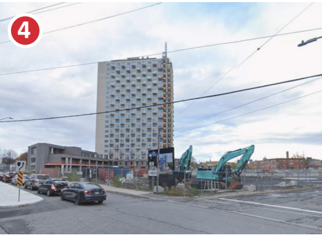
Looking north towards subject site
