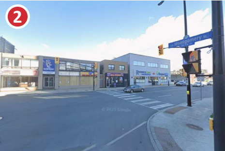
Looking North towards Montreal Rd.
