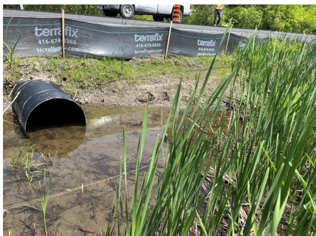
Photo 21 Facing north at existing conditions at Reach 3 and culvert at Marchurst Road, June 3, 2025.
