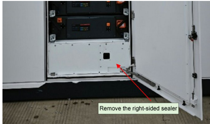
figure 5-28 Right Sealing Plate
