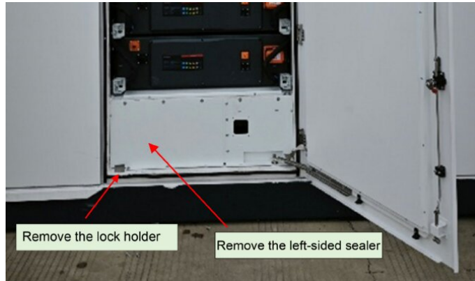
figure 5-30 Positions of Lock Holder and Left Sealing Plate
