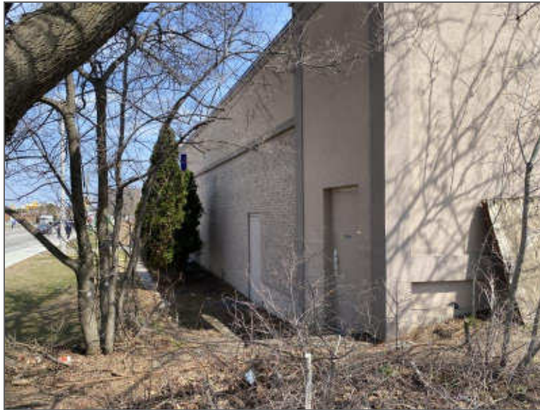
Photo 3 – Building A- northwest corner- looking east.
