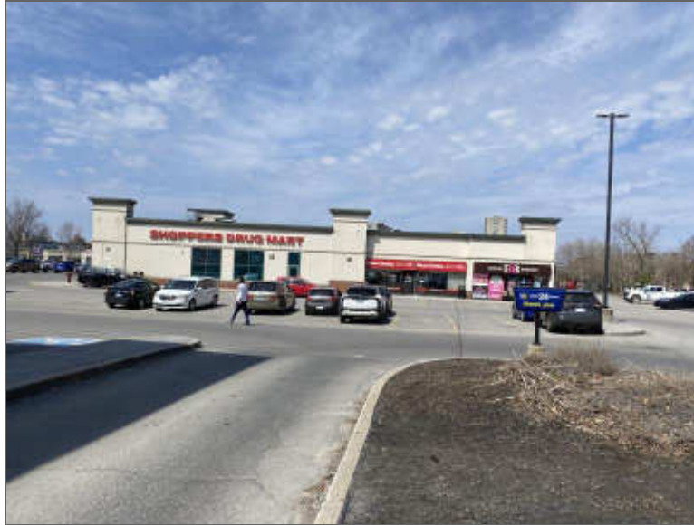
Photo 7 – Southeast corner of Site, looking north.
