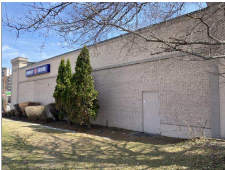
Photo 2 – View of Building A, north side, looking southeast.
