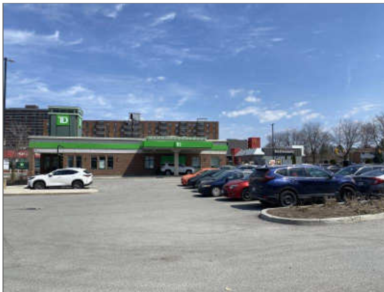
Photo 4 – View of Building B, looking east.
