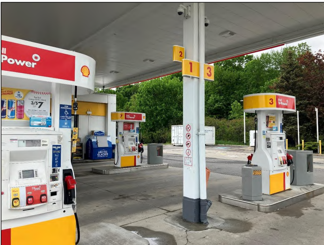
Photograph 4: View of pump islands, looking to the west.
