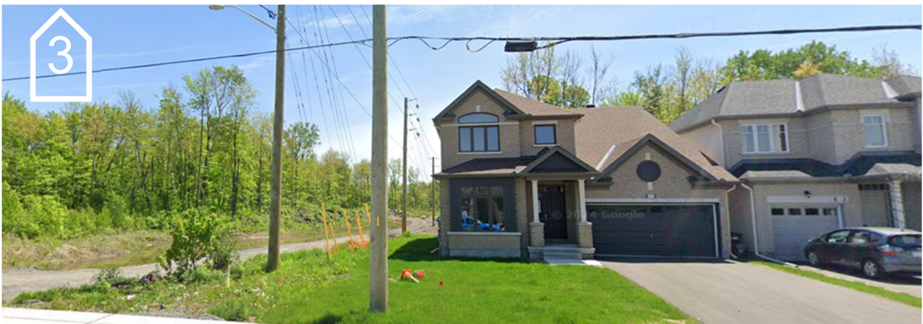
Figure 5: View looking south on Renaud Road
