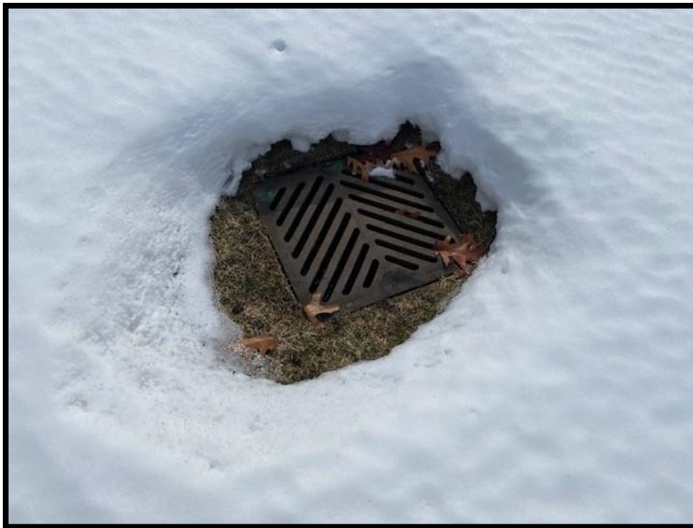
Photograph 6: View of the catch basin located in the central portion of the Phase I Property
