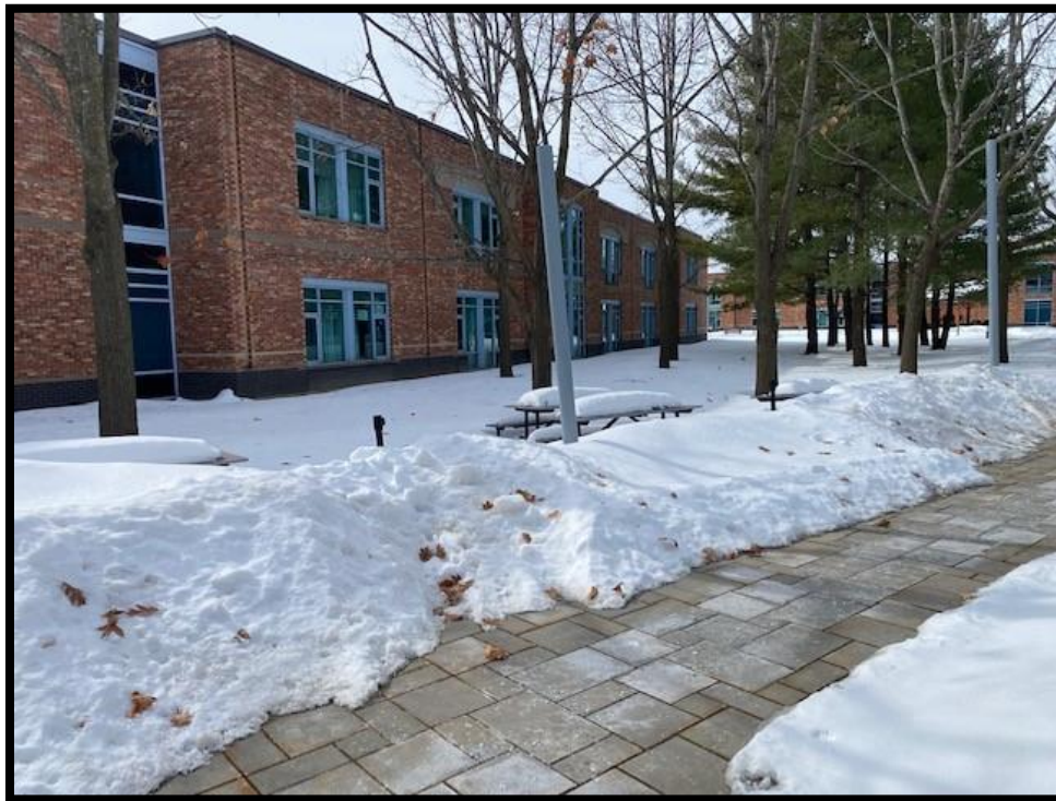
Photograph 2: View of the northeastern portion of the Phase I Property, facing south.
