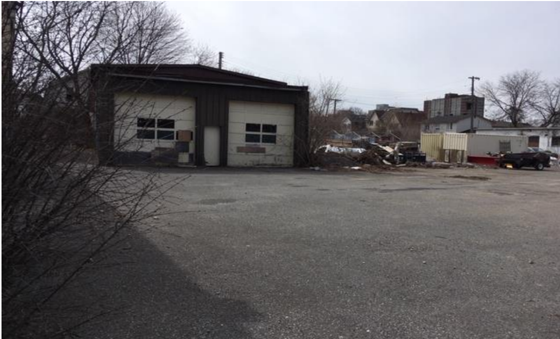
Photograph 5: Northeastern view of the Phase I Property, looking southwest.
