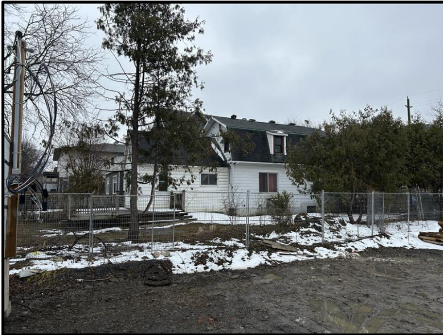
Photograph 5: View of the northern elevation of the 339 Roosevelt Avenue dwelling.
