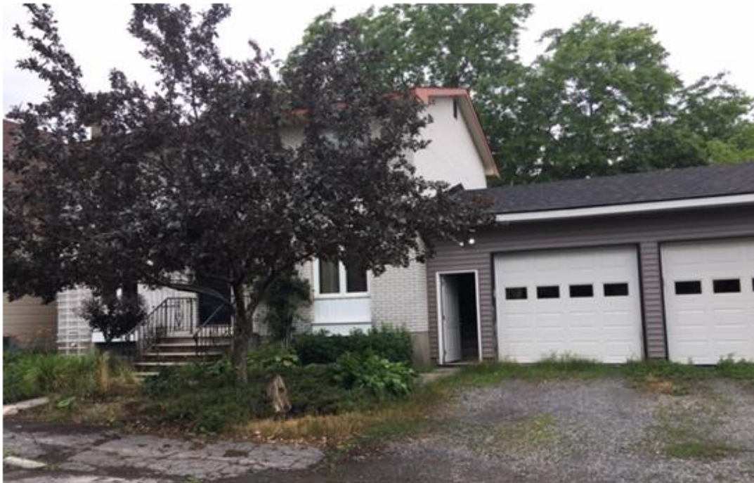
Photograph 14: Residential dwelling at 344 Winston Avenue, situated on the southwestern portion of the Phase I Property, west.
