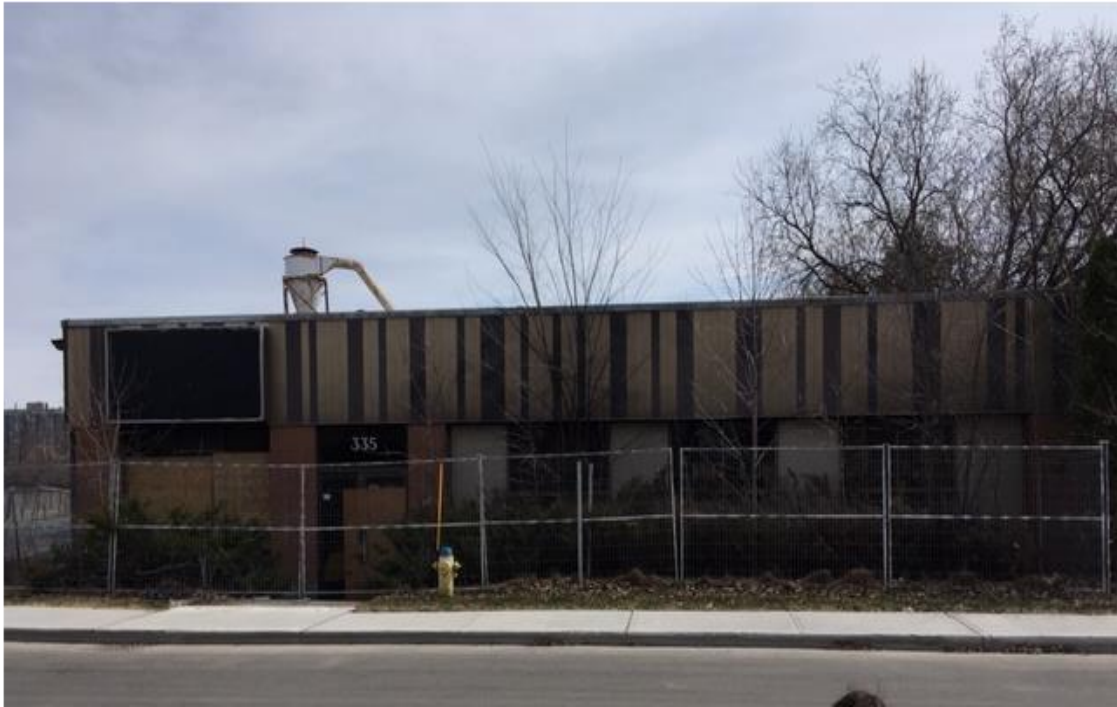
Photograph 1: West view of the Phase I Property, taken from Roosevelt Avenue looking east.
