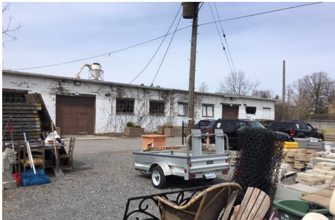
Photograph 12: Central west view of the Phase I Property, taken from the central south side of the site, looking northwest.
