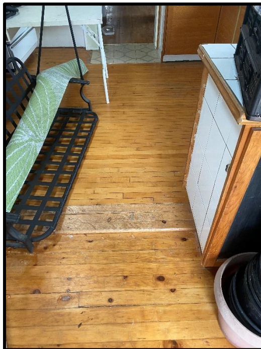
Photograph 6: View inside the 339 Roosevelt Avenue dwelling.
