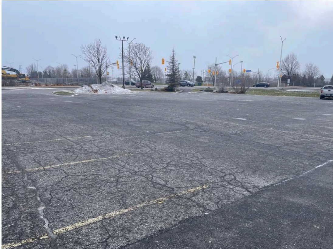
View from site facing southwest
