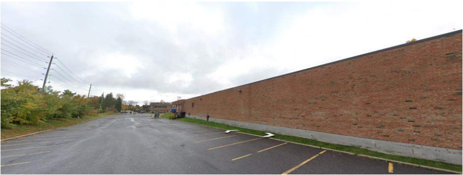
View 4: Looking East
