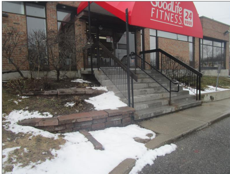
Photo 3 – Site Building (east elevation).
