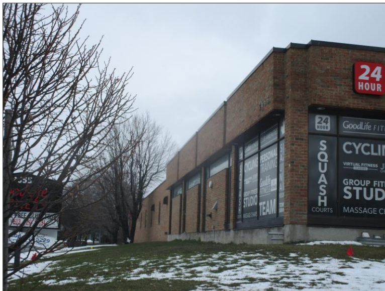
Photo 2 – Site Building (south elevation).
