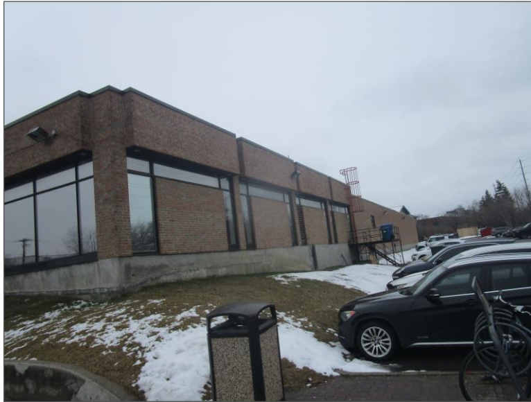
Photo 1 – Site Building (north elevation).
