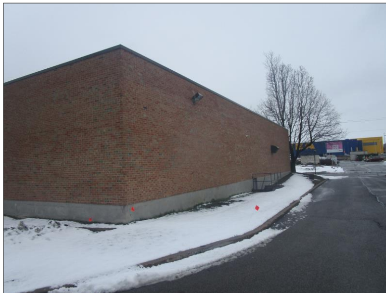
Photo 4 – Site Building (west elevation).
