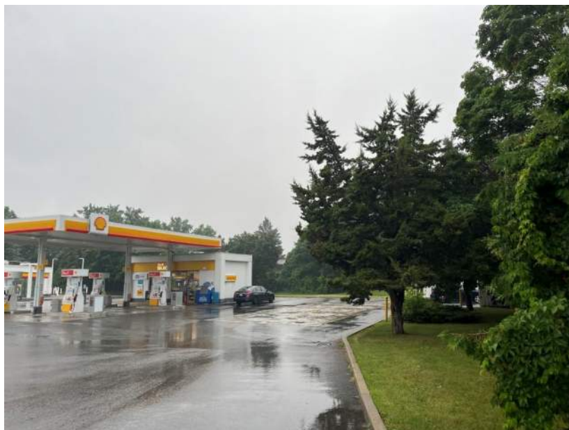
Photograph 2: North property boundary along Katimavik Woods. Existing fuel pumps and kiosk to be removed. Direction: West
