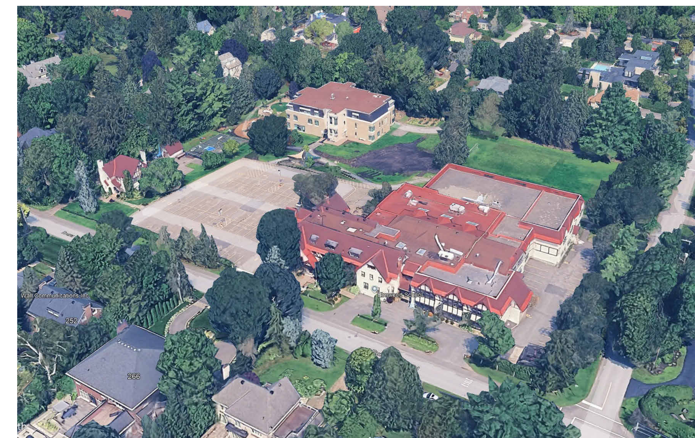
AERIAL VIEW OF EXISTING SITE AND BUILDINGS
