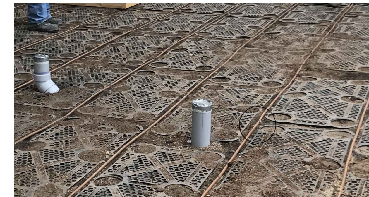
DRIP LINE PRECEDENT AT SILVA CELLS
