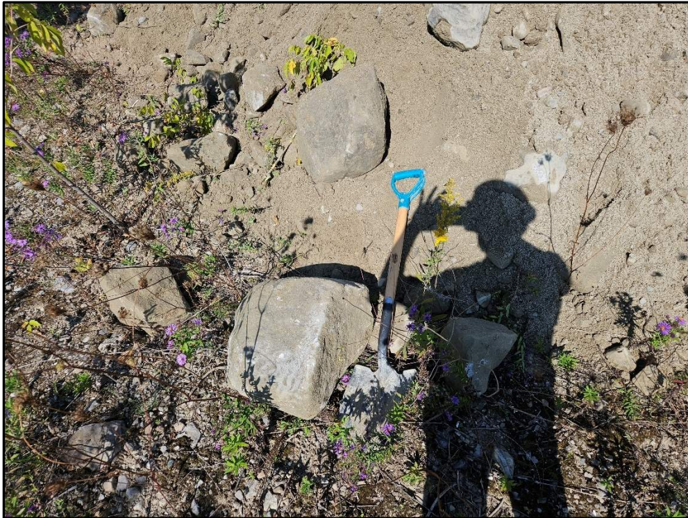
Photo 11: Photo illustrating the boulders excavated from the test pit TP 7-24.
