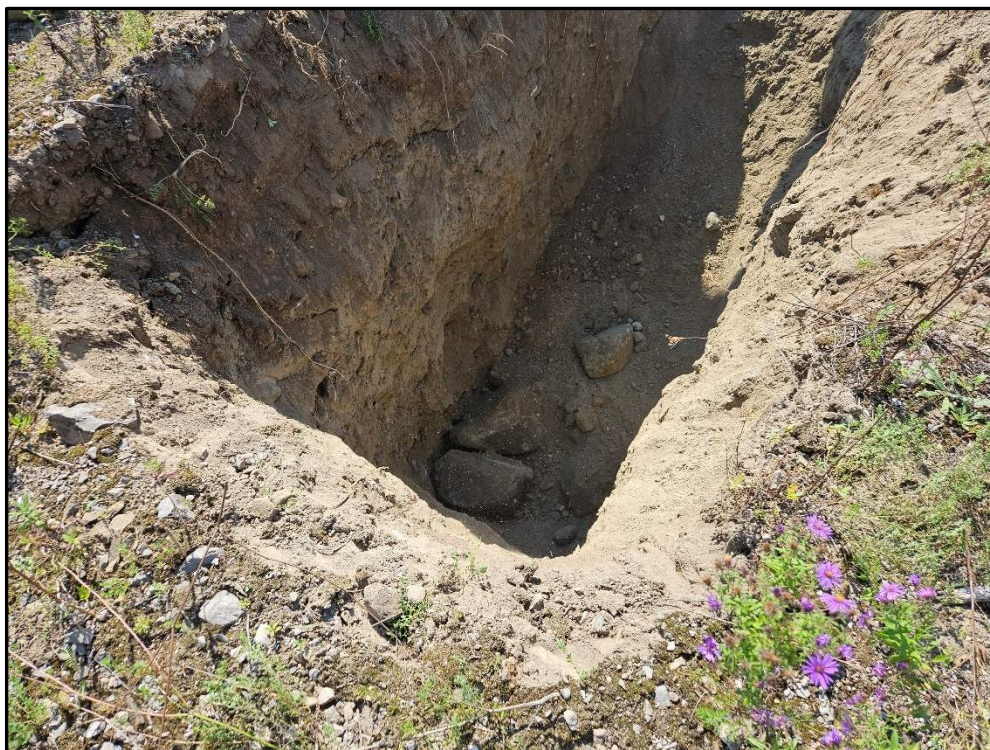
Photo 12: Photo of the test pit TP 7-24.
