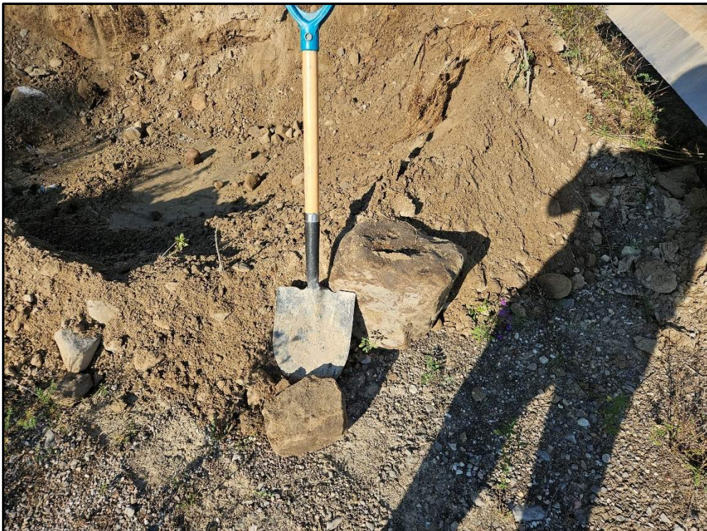
Photo 4: Photo illustrating the boulders from the test pit TP 2-24.
