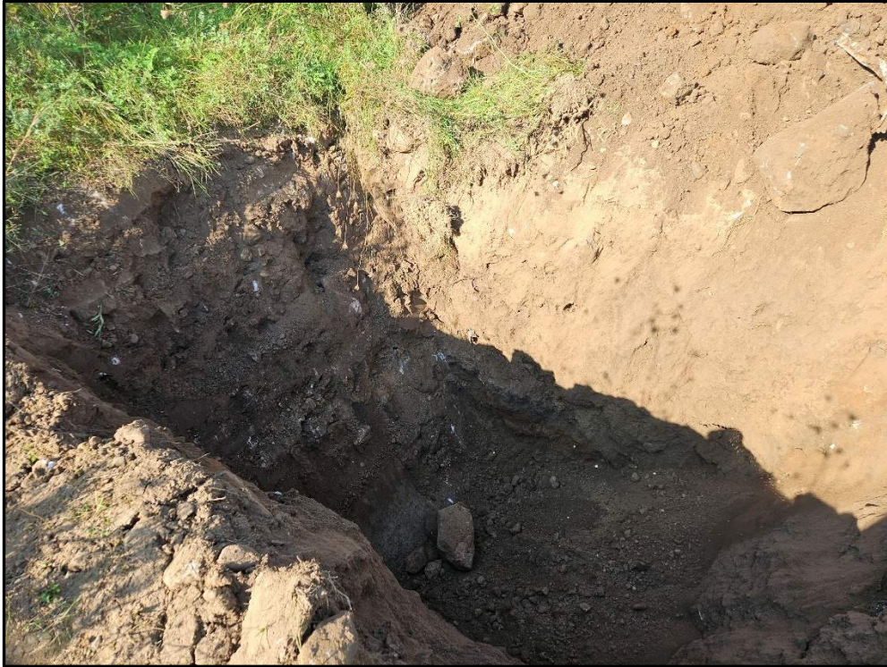
Photo 3: Photo of the test pit TP 2-24.
