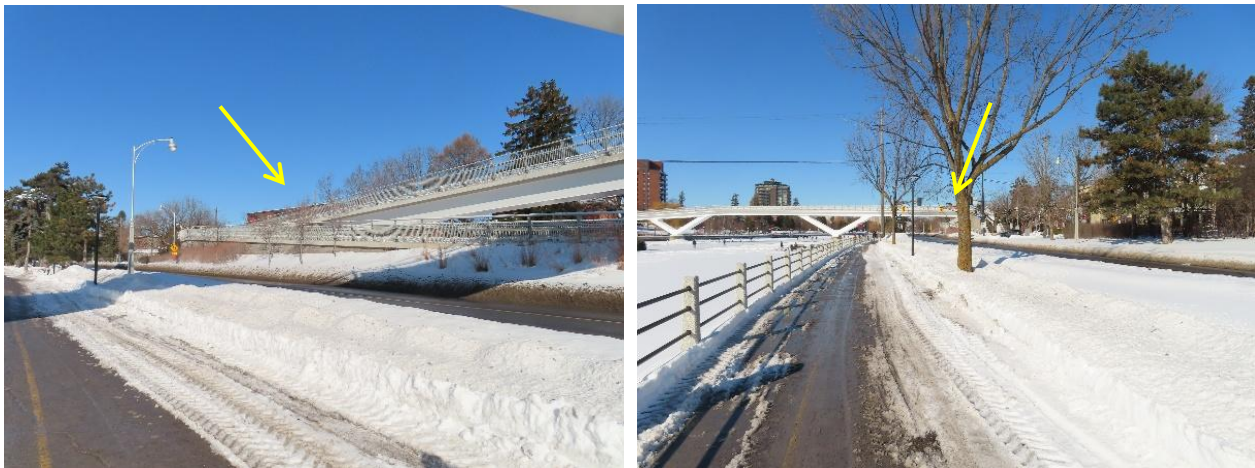
Figure 8: Views of the existing property obscured by the Flora Footbridge, photographed from the East side of the Canal (Source: Juxta Architects)
