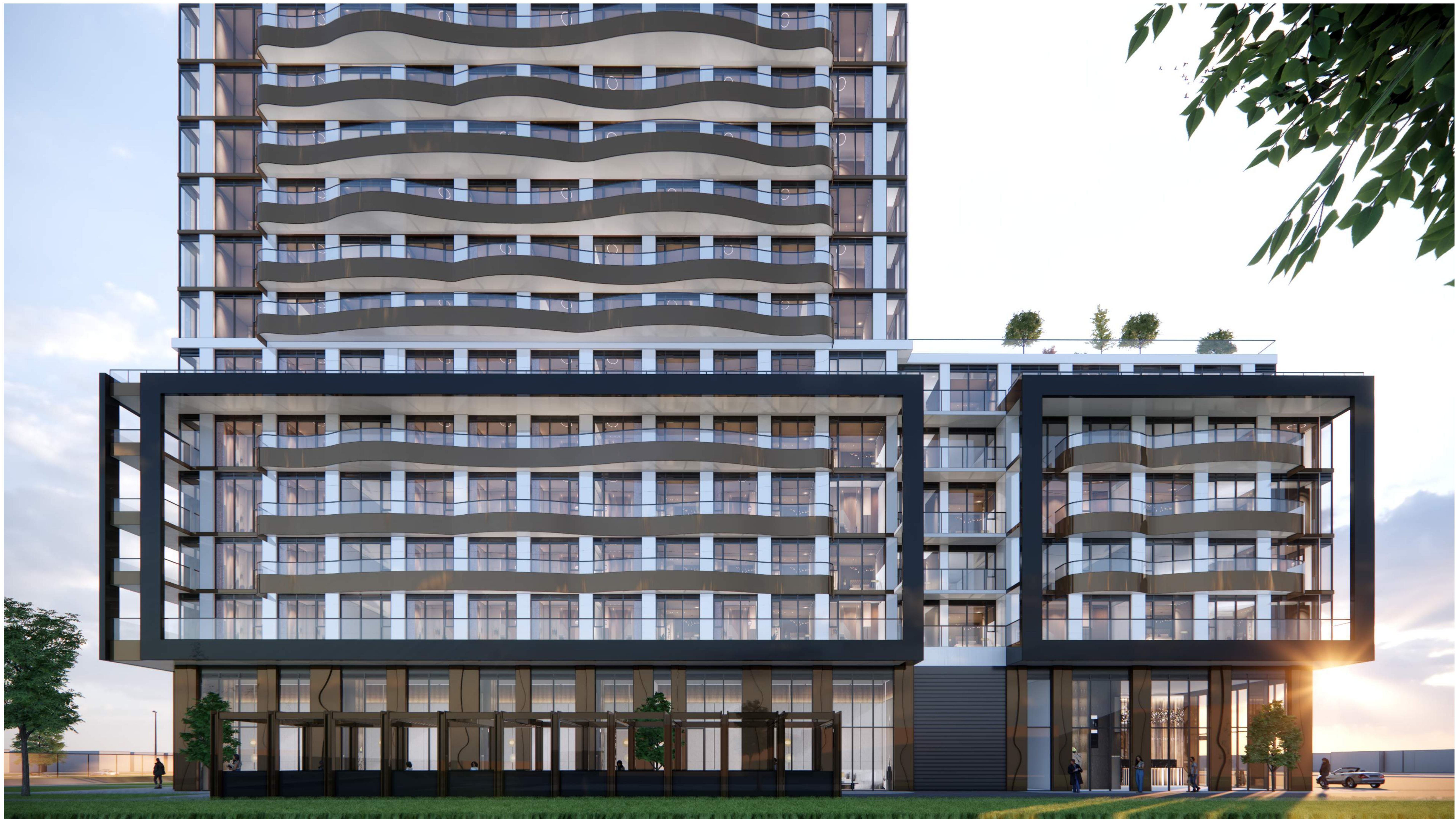
VIEW LOOKING WEST FROM EXISTING 6-STOREY OFFICE BUILDING
