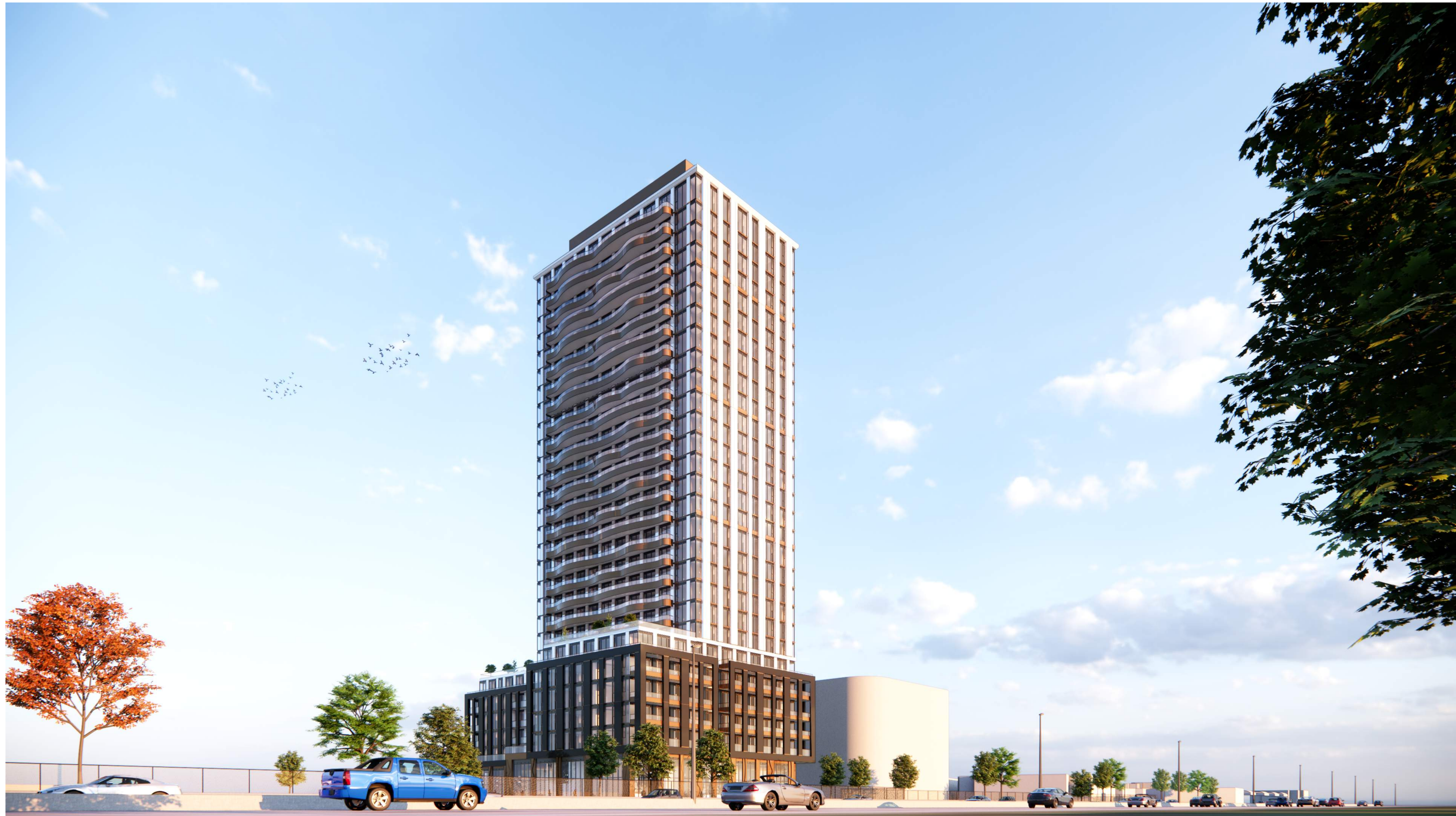
VIEW FROM TRANS-CANADA HWY LOOKING NORTH EAST
