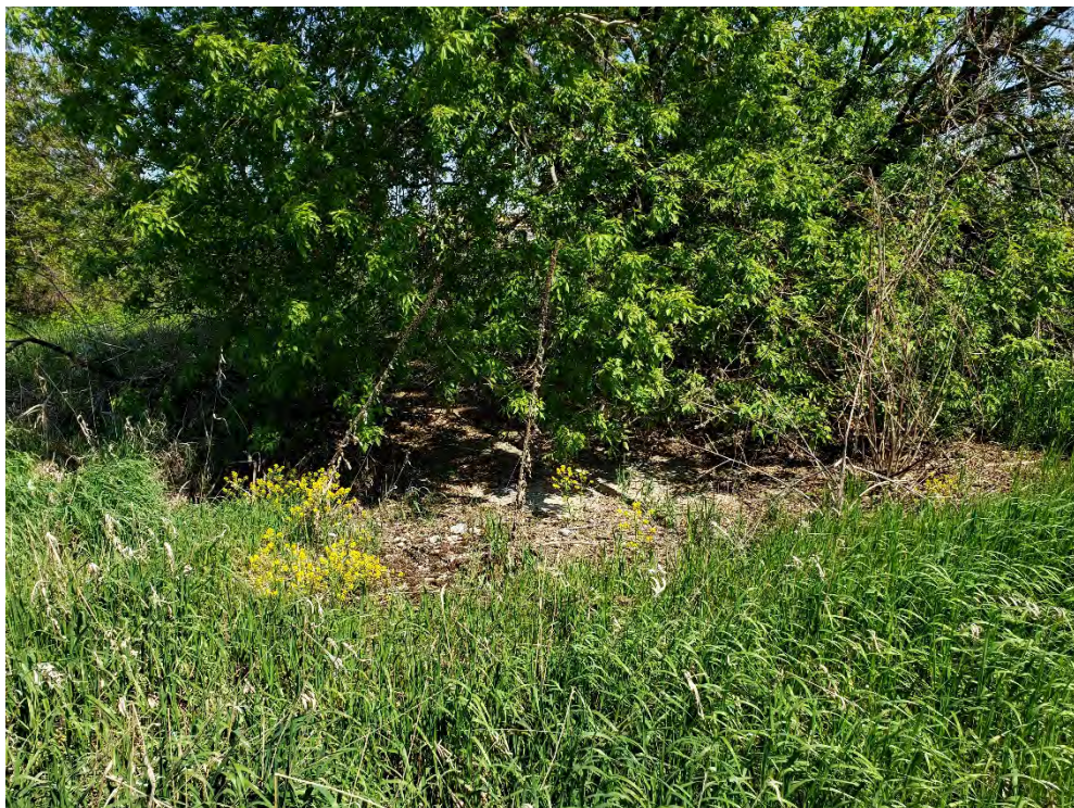
Image 6: Concrete floor of former northern outbuilding, view north.
