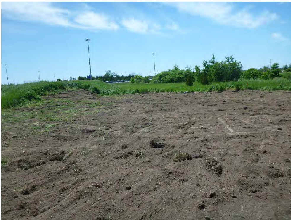
Image 48: Operation 2 backfilled following MTR, view west.
