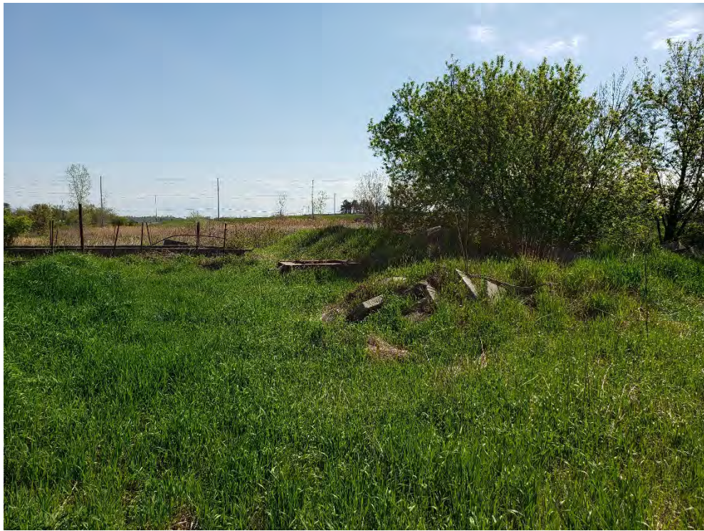
Image 5: Mounds of displaced soil and structural material south and west of former dairy barn, view east.
