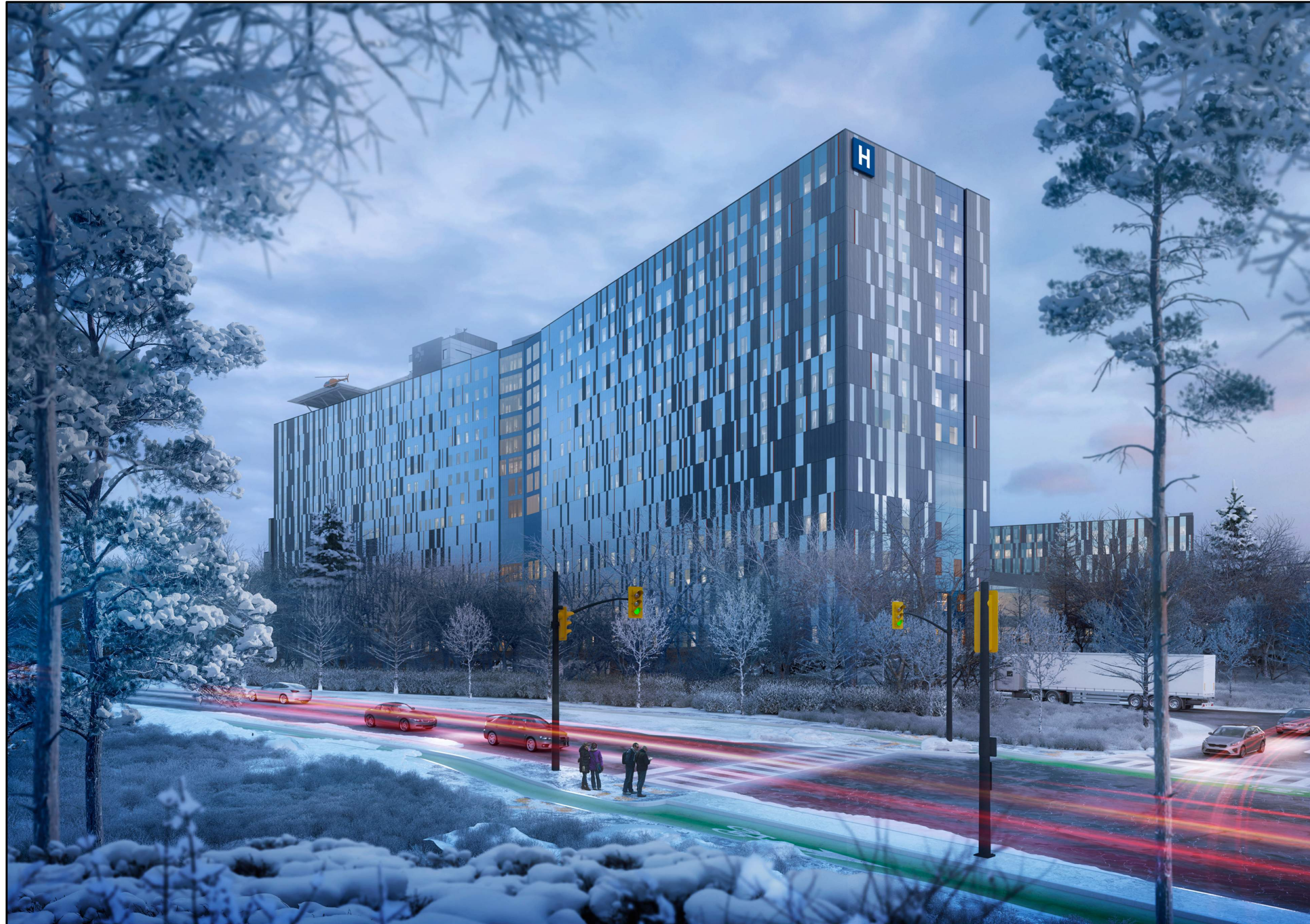
View 6: View of the Facility from the intersection of Prince of Wales Drive and Road B at grade - Winter View
