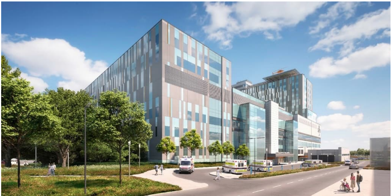
Plate 6: View of the proposed southwest corner facades as seen at grade from Road E looking north.
