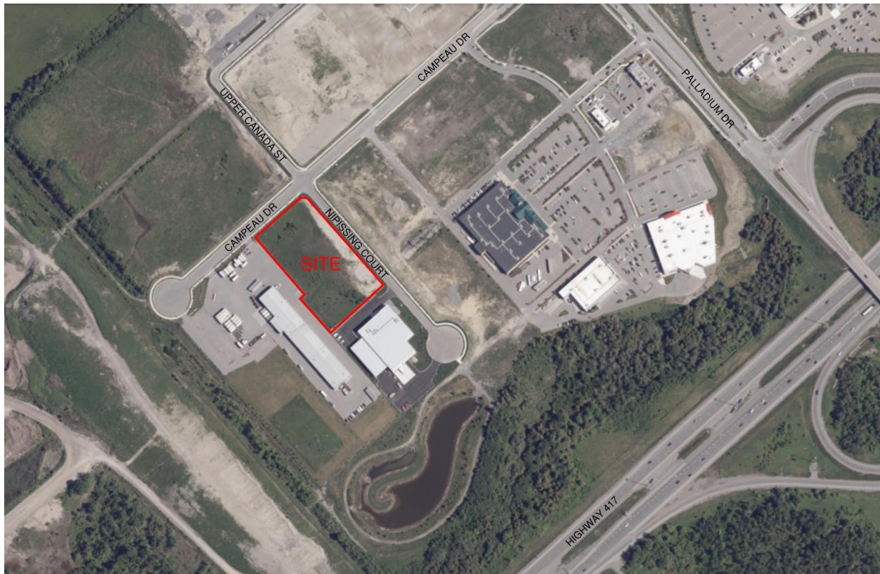
Figure 1 – Aerial View of the Subject Site
