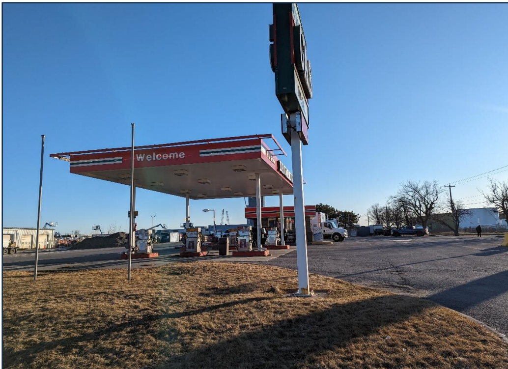
Photograph 6: View looking east at 1925 Merivale Road – March 21, 2025.
