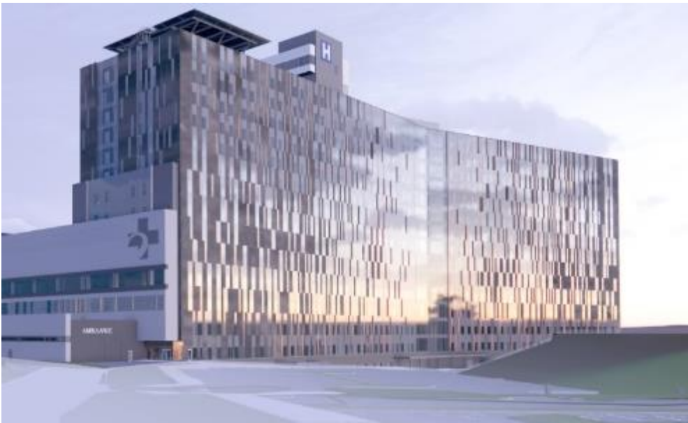
Figure 2.2-2: Rendering demonstrating reflectivity of porcelain panels and glazing
