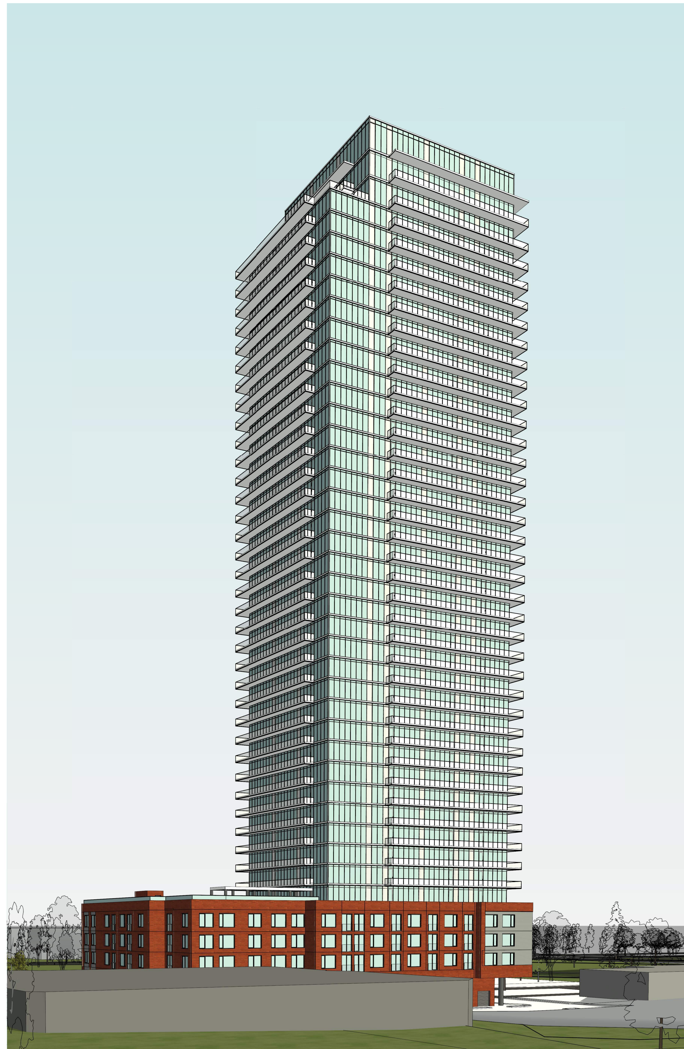
VIEW LOOKING SOUTH-EAST
