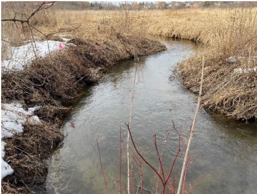
Toe erosion at the Poole Creek between cross-sections A and B
