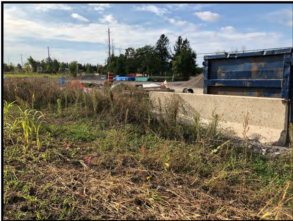
Figure 2: Barriers and dumpster along the western edge of the Morgan site, by unit 585E 305N (MH1037-D016).
