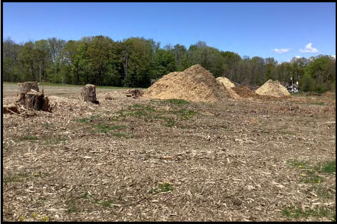
Figure 25: Wood chips and mulch pile at 1070 March Rd (D01).
