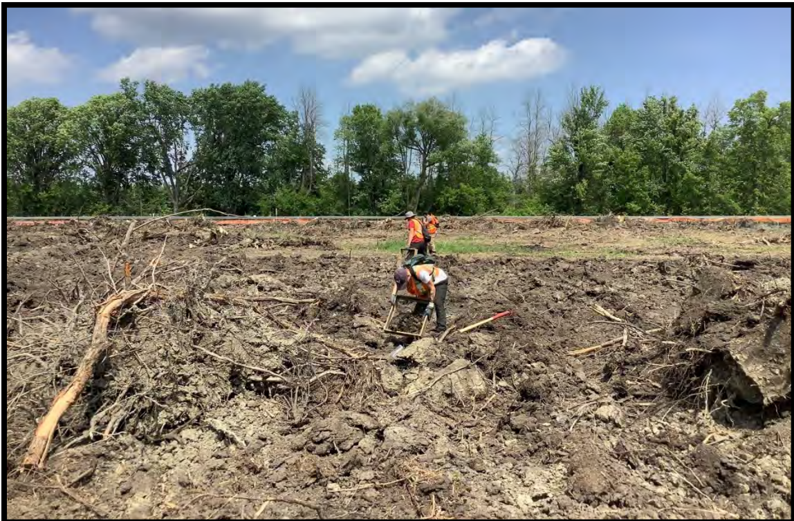
Figure 12: Testing through disturbed soils from tree grubbing, note the exposed subsoil (D112).
