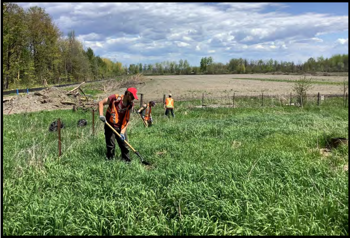
Figure 31: Testing slope behind 1070 March Rd (D06).
