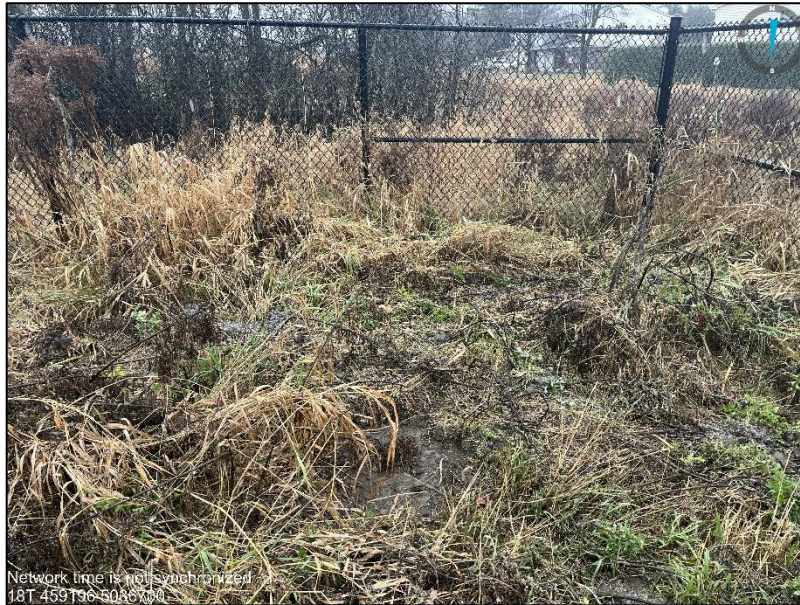
Municipal storm sewer manhole observed in the southwest portion of the Site
