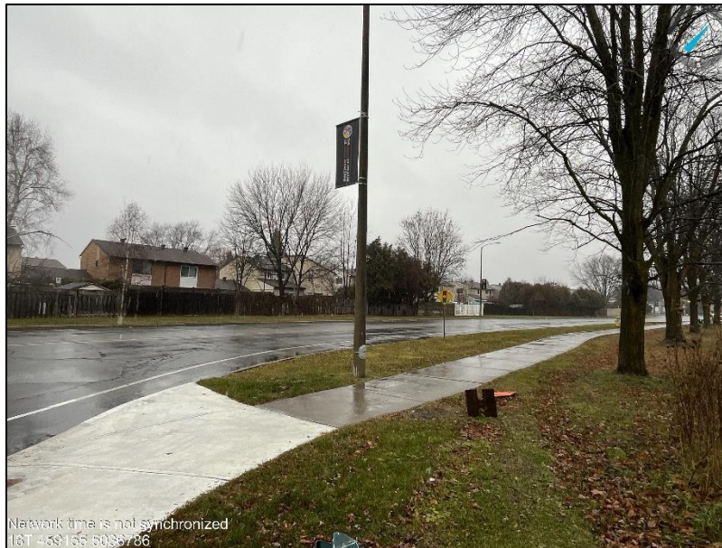
North adjacent residential properties
