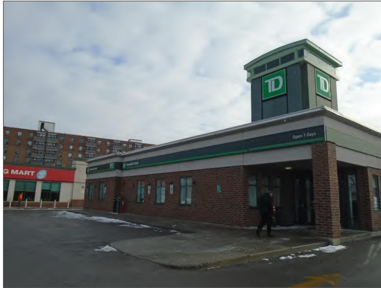
Photo 1 – Site Building B (northwest elevation).
