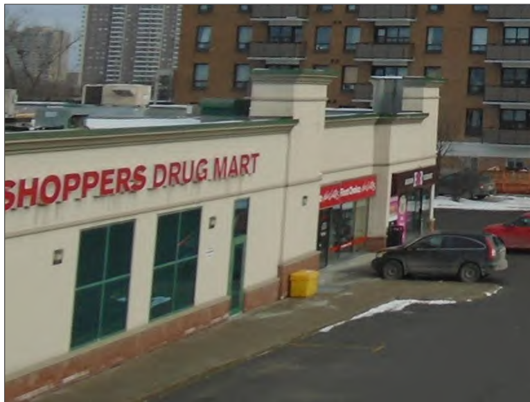
Photo 4 – Site Building C (southwest elevation).
