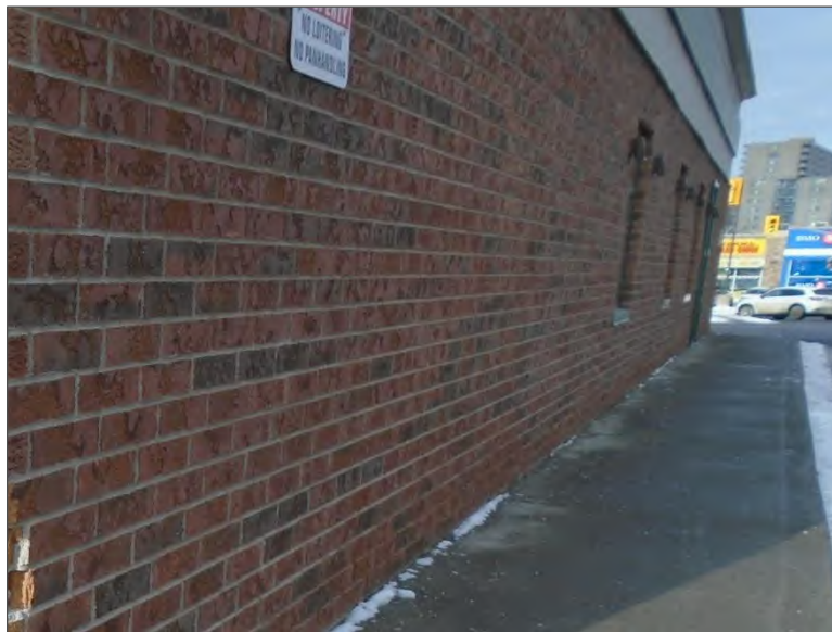
Photo 2 – Site Building B (northeast elevation).
