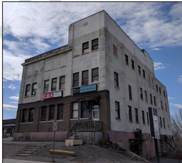
Photo 1: 951 Gladstone Avenue, south and east elevations [JCAL 2018].
