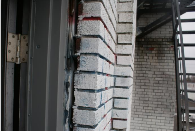
Figure 32: View of the exterior brickwork from a second-floor fire escape. Note the highly textured brick surfaces and recessed joint profile. Source: Commonwealth 2021.
