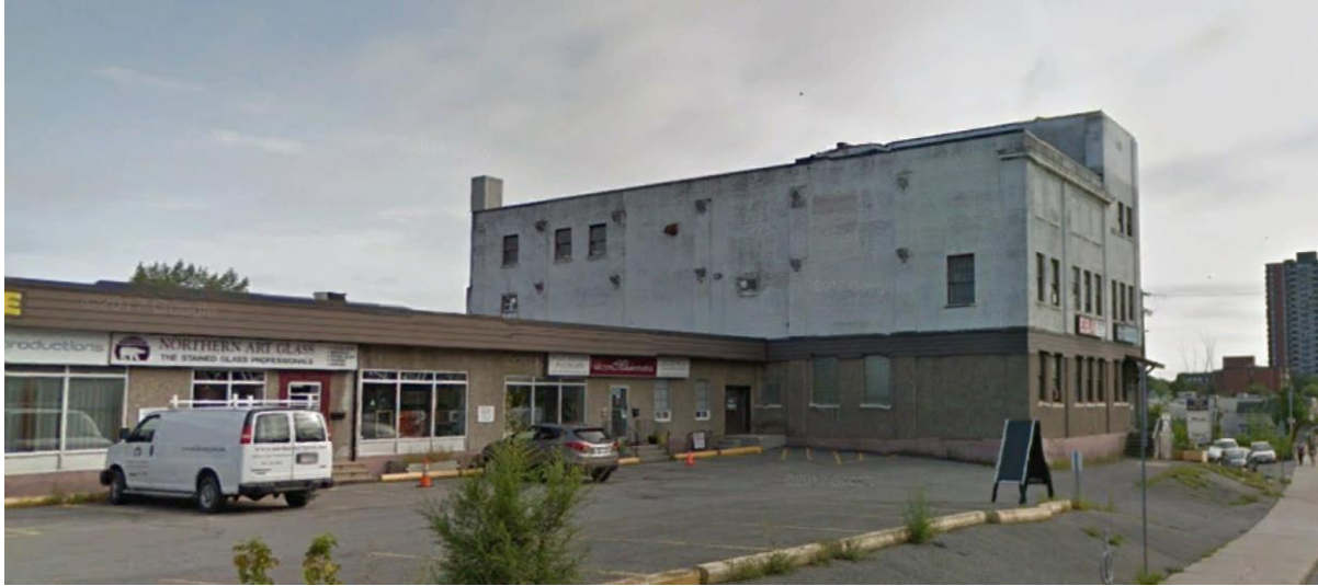
Figure 4: View of the west side of the former Standard Bread Company factory. Note the grade change between the first-floor level and the sidewalk along Gladstone. Source: Google Earth.
