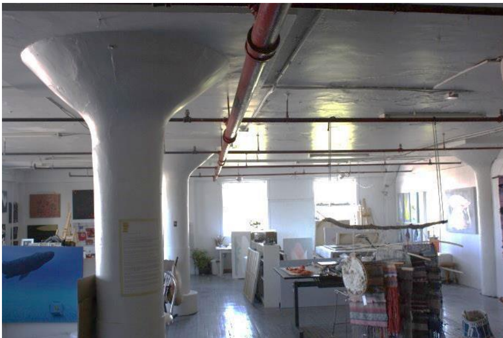
Figure 10: Interior view of the mushroom columns. Source: Commonwealth 2021
