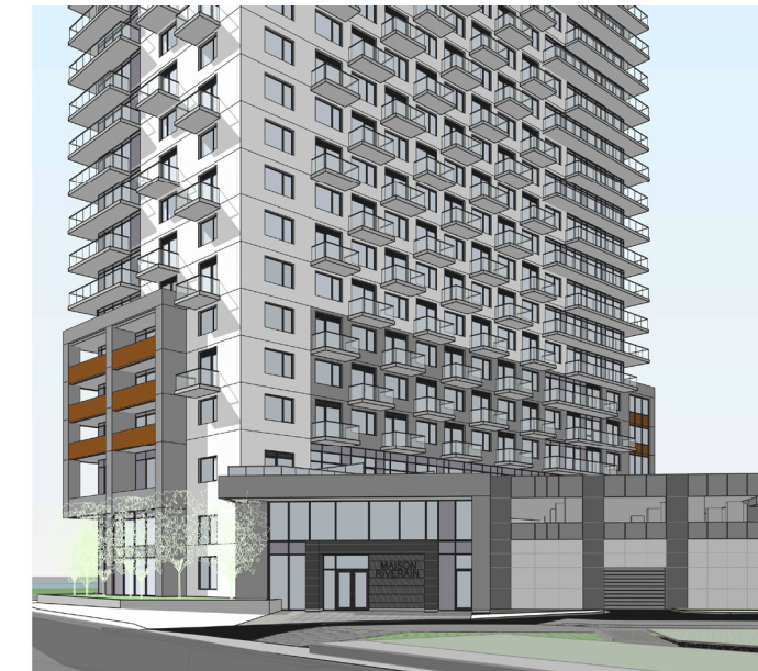
View from internal road - Looking at main entrance
