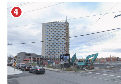
Looking north towards subject site
