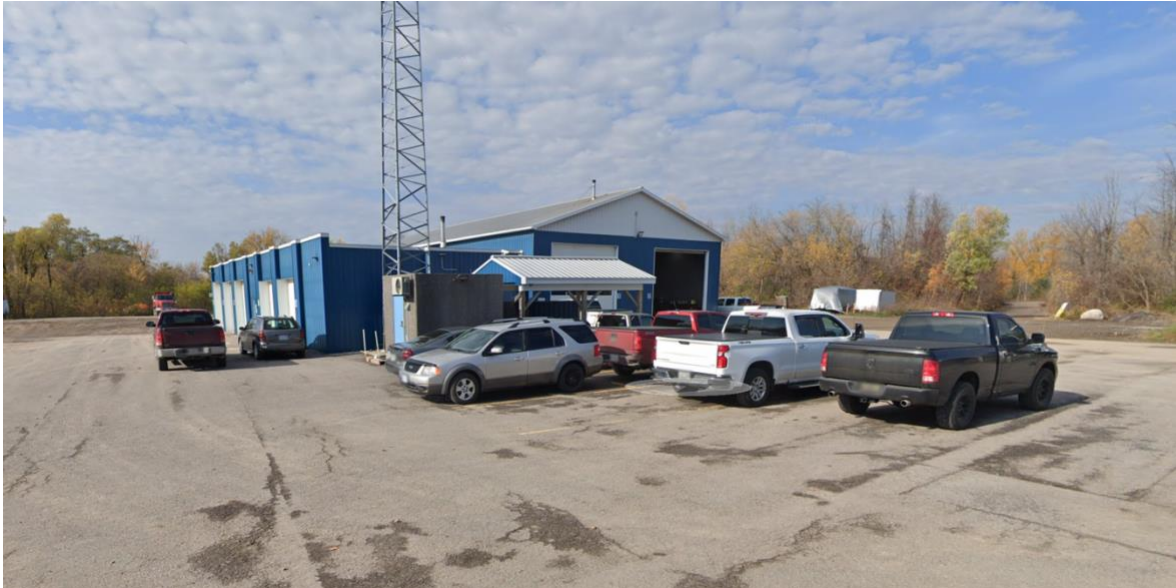
Figure 6: Existing buildings and parking on the subject site, looking east
