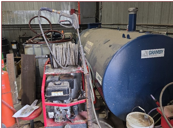
Photograph C1 – Looking southeast at an AST and tote.
