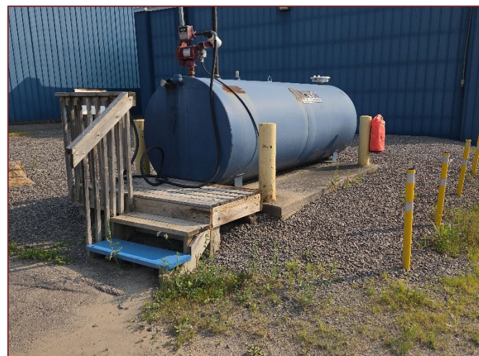
Photograph C4 – Looking north at a diesel fuel AST on a concrete pad.
