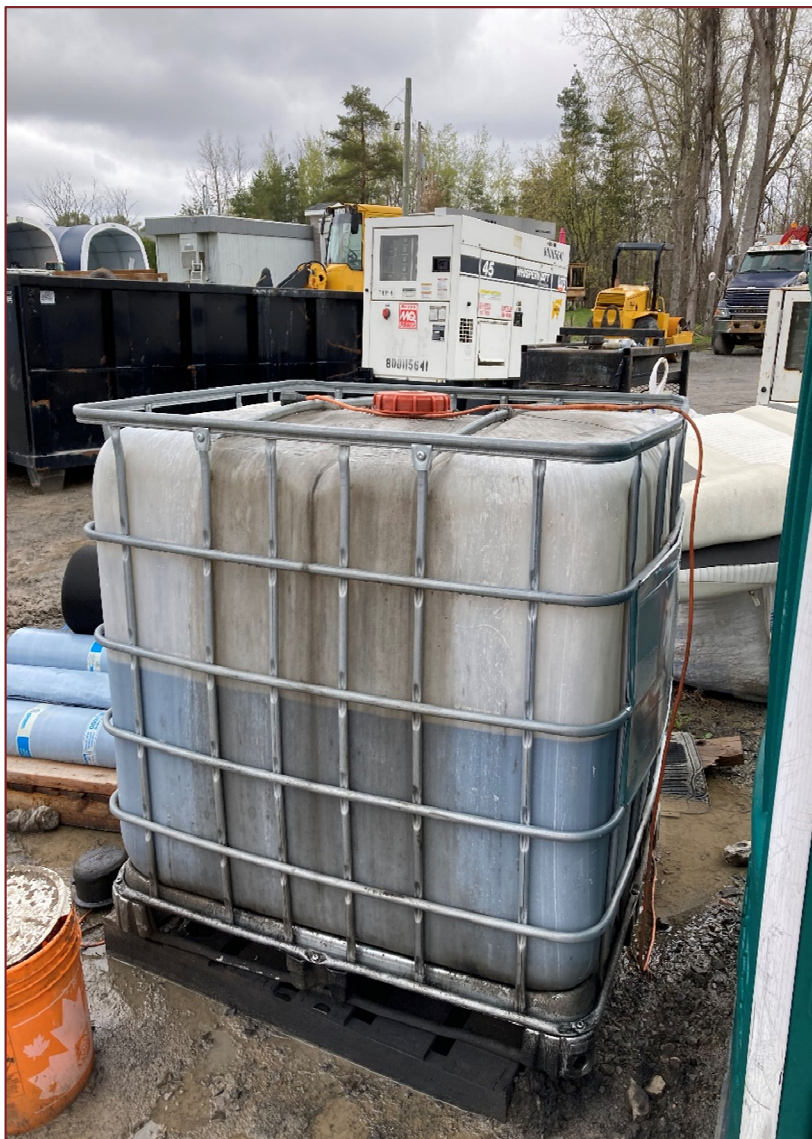
Photograph 27: Tote containing waste oils from CACE construction.
