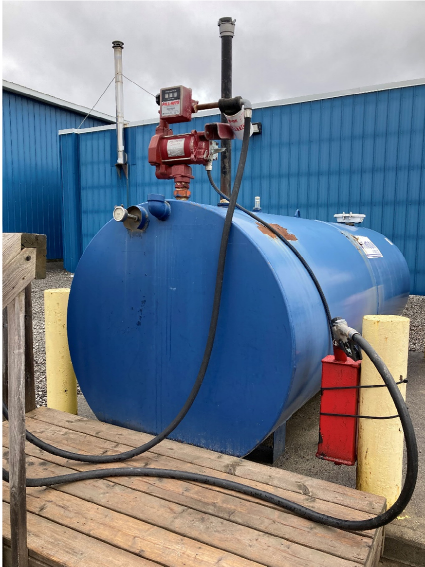
Photograph 7: 1000 Liter double walled coloured diesel storage tank from 2013
